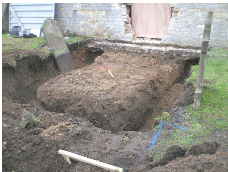
Plate 2 – The excavated foundation trenches, looking southeast
