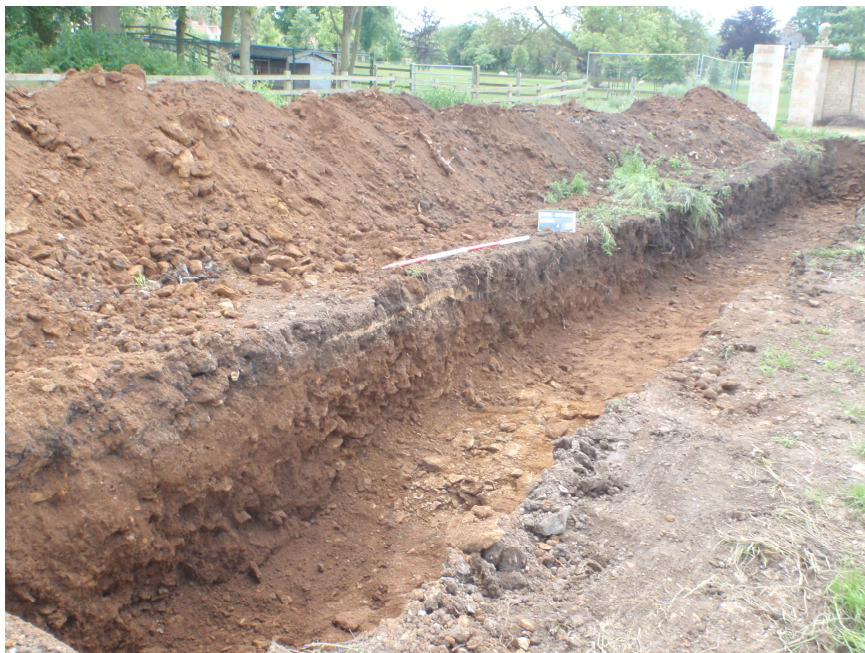
Plate 5 – Section 1, looking southeast
