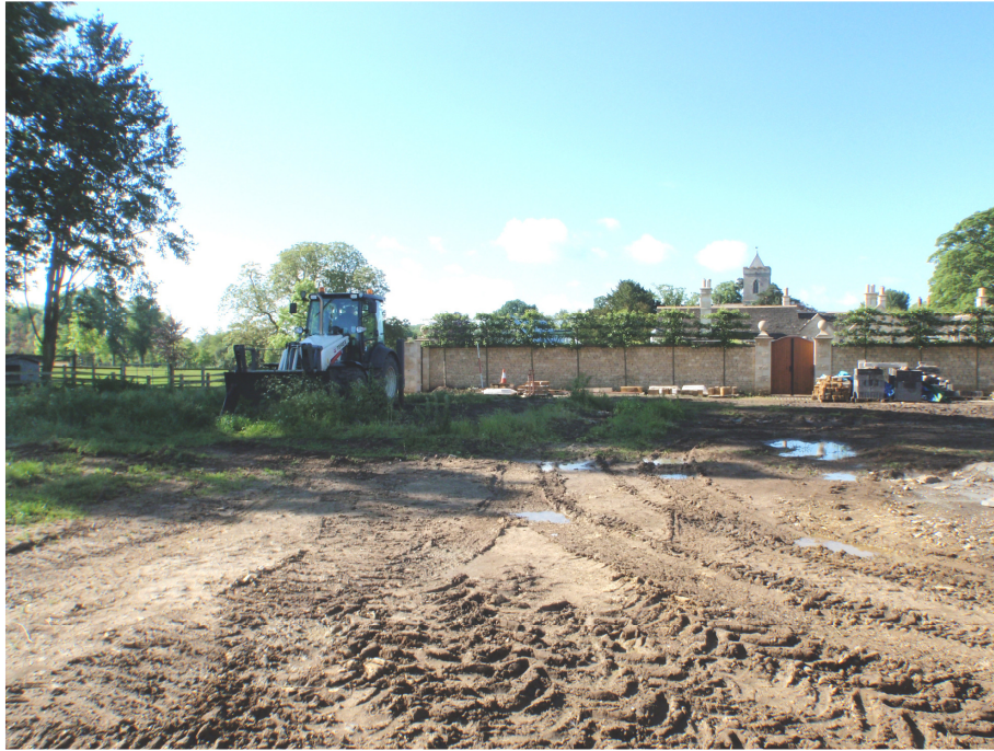
Plate 1 – General view over the area of the proposed tennis court with the Old Hall in the background, looking south
