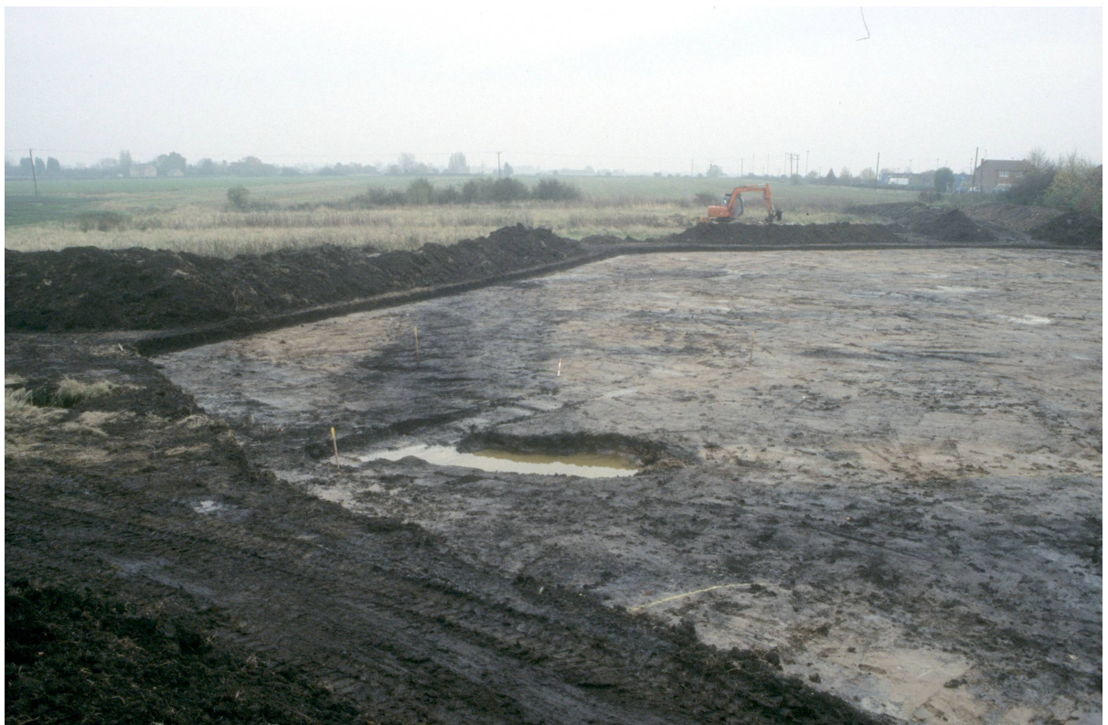
Plate 6. Pre excavation view of northern, turbine, area of site looking east
