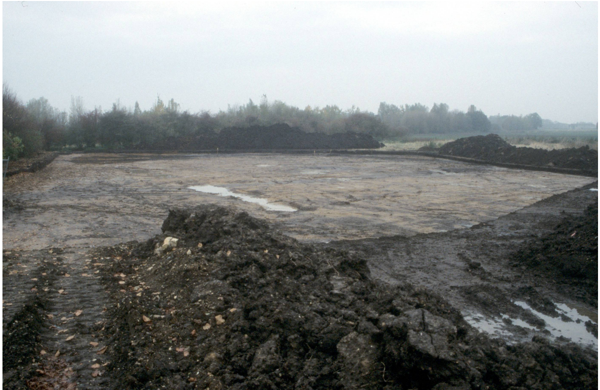
Plate 3. Pre- excavation view of site looking west, 1 st November 2004
