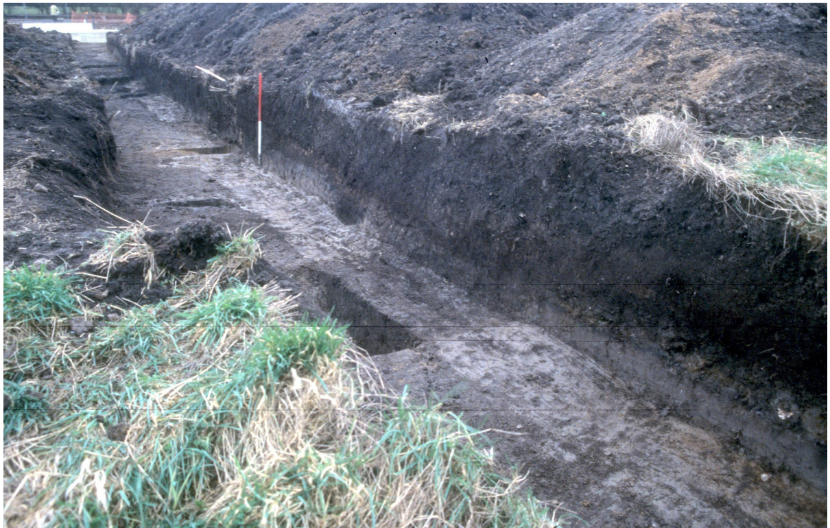
Plate 24. Overall view of pipe trench, Section 212, looking southwest, 17 th January 2005
