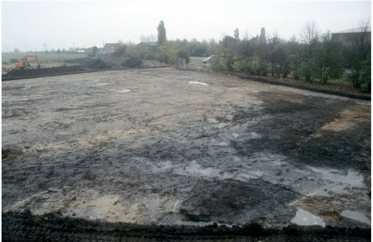
Plate 5. Pre-excavation view of site looking ESE
