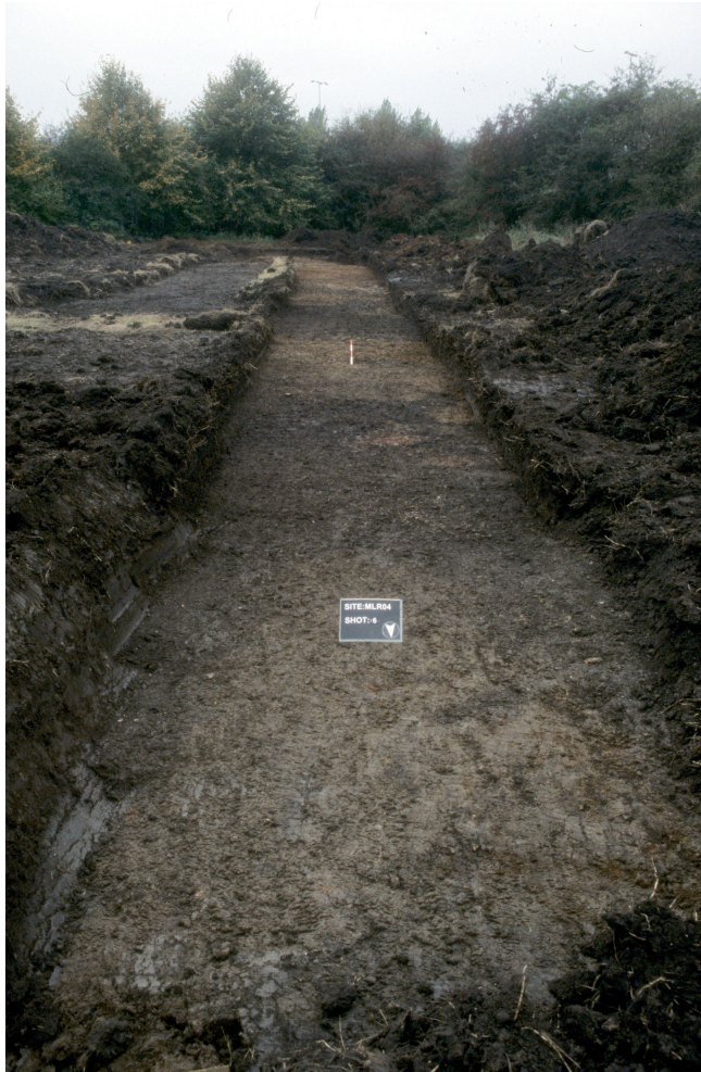
Plate 1. Pre-excavation view of service trench looking south, 19 th October 2004
