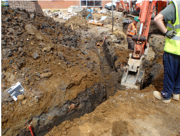
Plate 7 – Section 9, looking north
