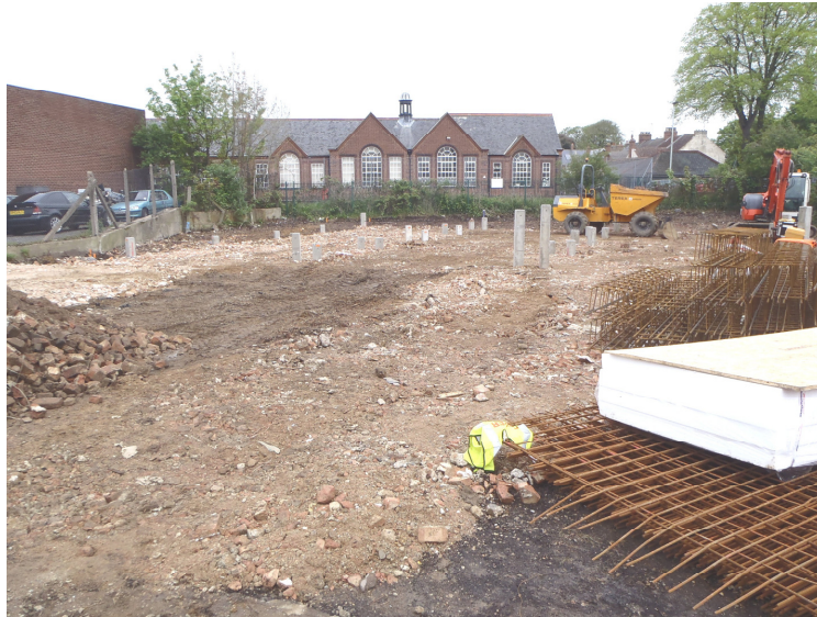
Plate 1 – General view across the site, looking northwest
