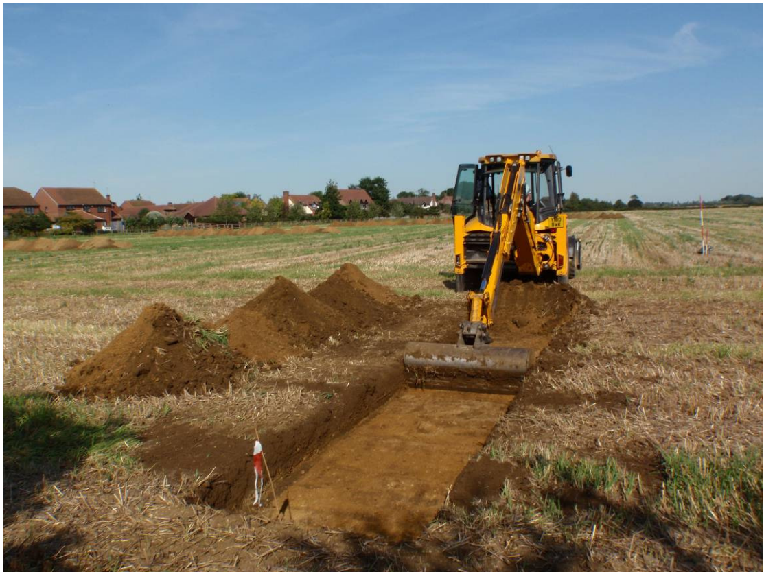
Plate 2. Machining Trench 7 looking east
