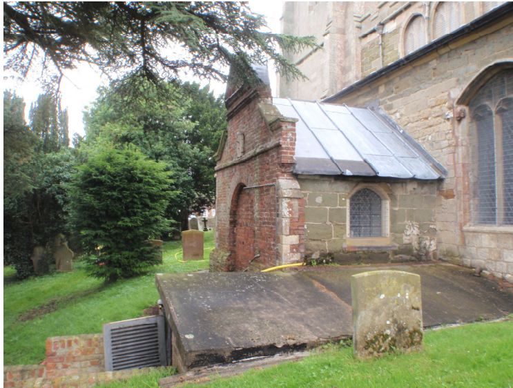
Plate 1 – General view along the route of the gas pipe, looking west
