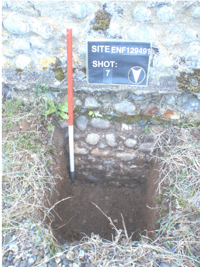
Plate 5 – Test Pit 6 showing the foundations of the chancel, looking south
