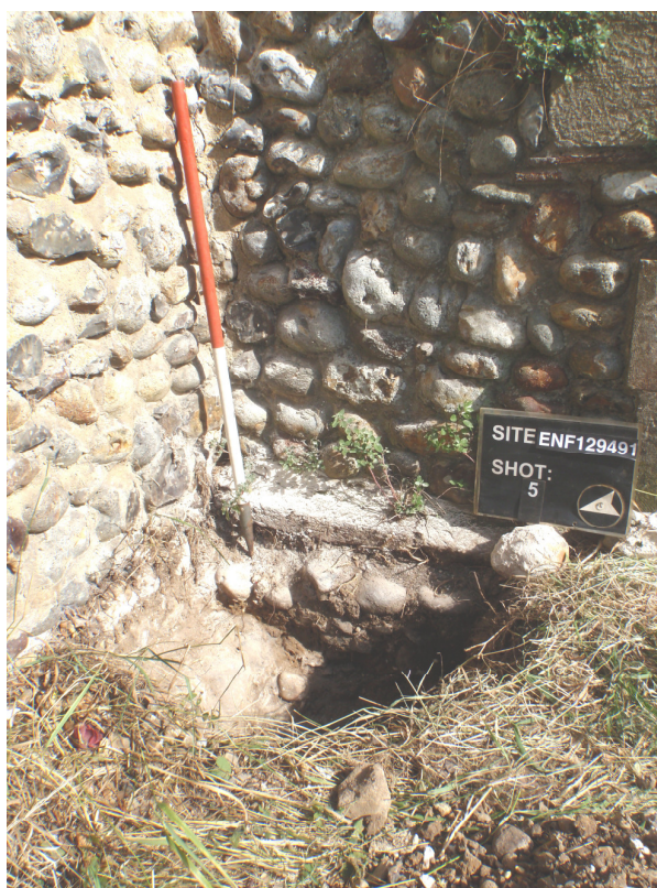
Plate 4 – Test Pit 4, earlier buttness overlying stepped foundations of the nave, looking northeast
