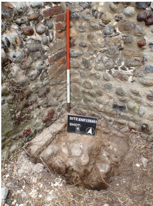
Plate 3 – Test Pit 3 showing the extent of the earlier buttness, looking northwest
