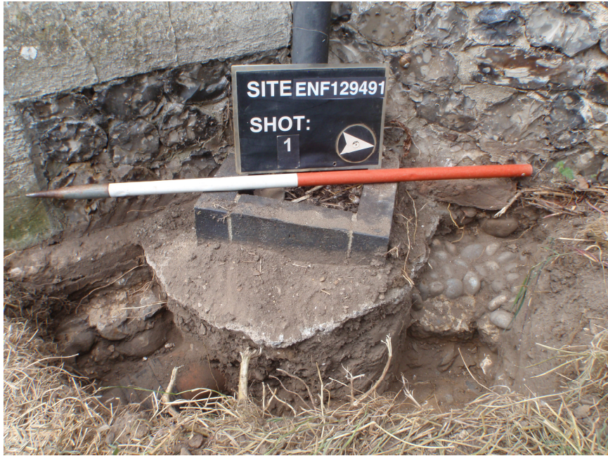
Plate 1 – Test Pit 1, showing the porch foundations, looking west
