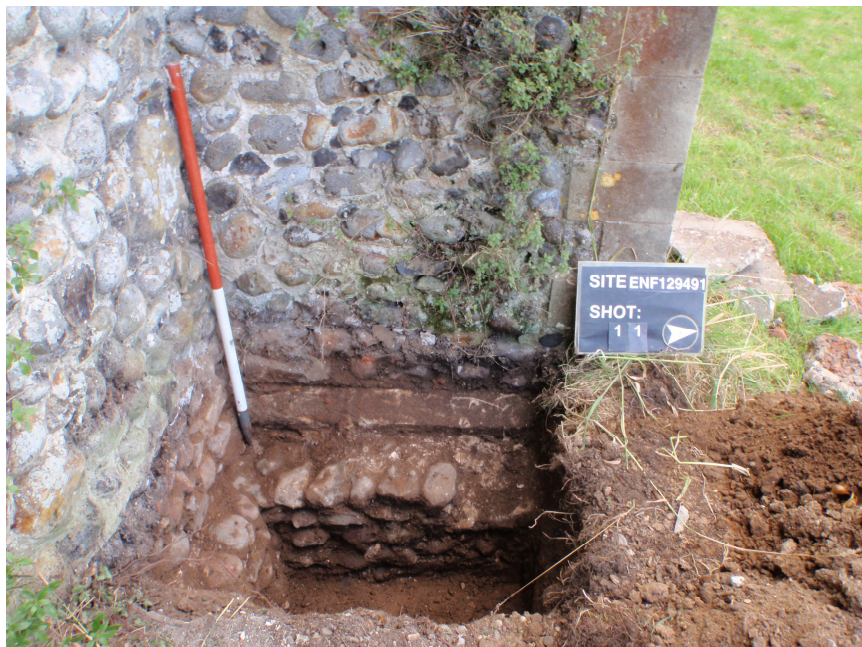
Plate 6 – Test Pit 8, stepped foundations of the church with the earlier and later buttresses built against it, looking west
