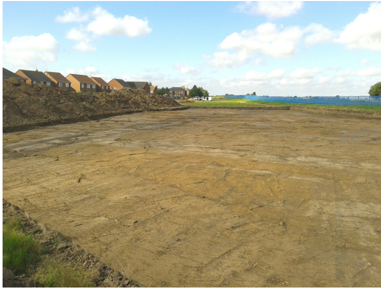
Plate 1 – General view of the site following initial stripping, looking southwest
