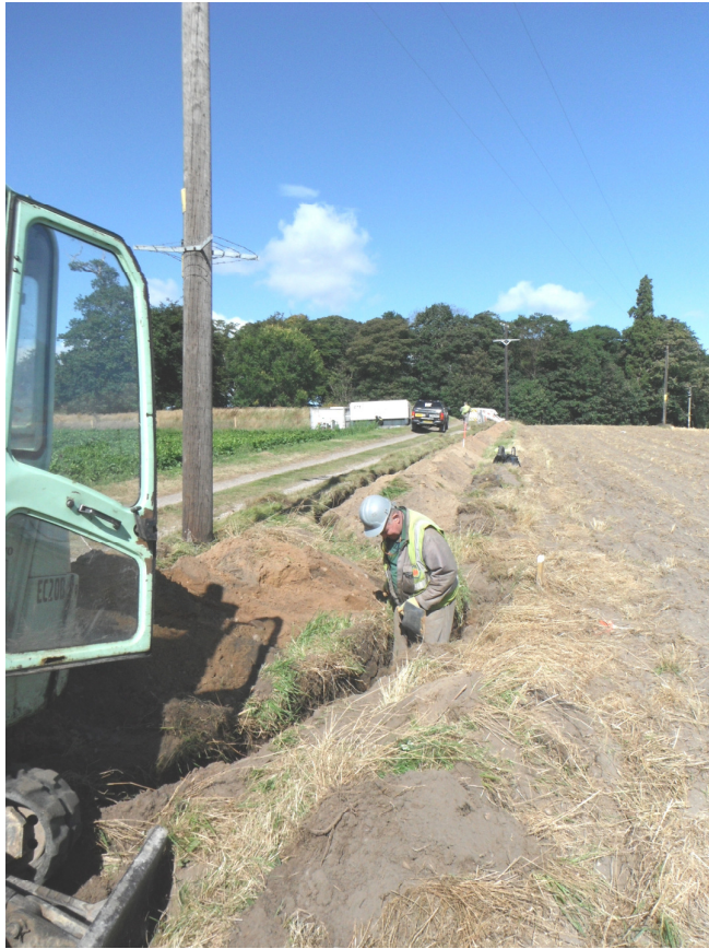
Plate 1 – General view looking north along the cable trench
