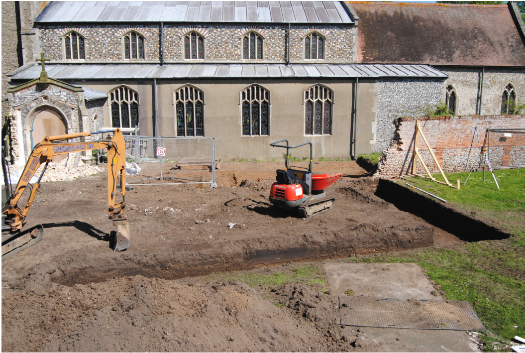
Plate 1 – View of St Andrew's church showing work in progress, looking north
