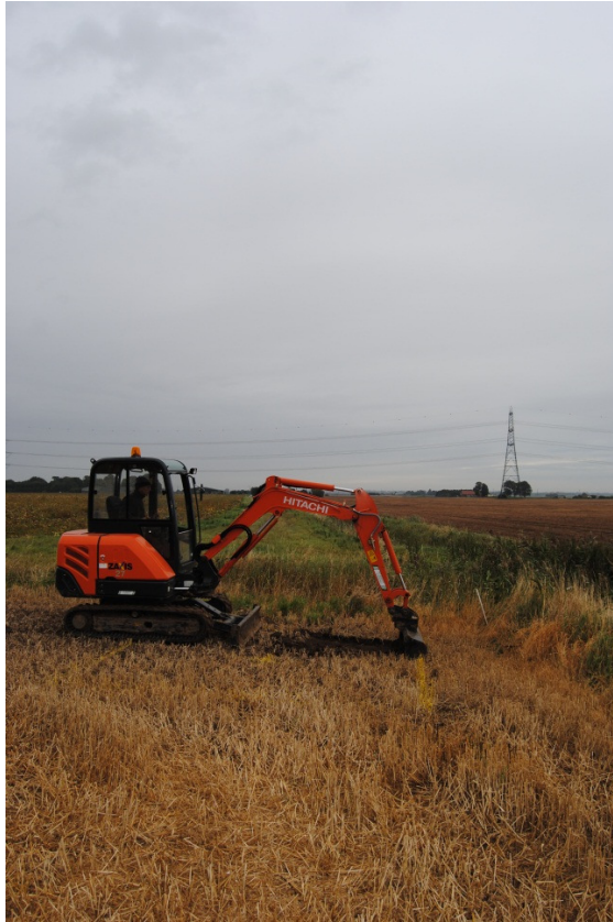
Plate 1 - Turbine Base A under excavation, looking east
