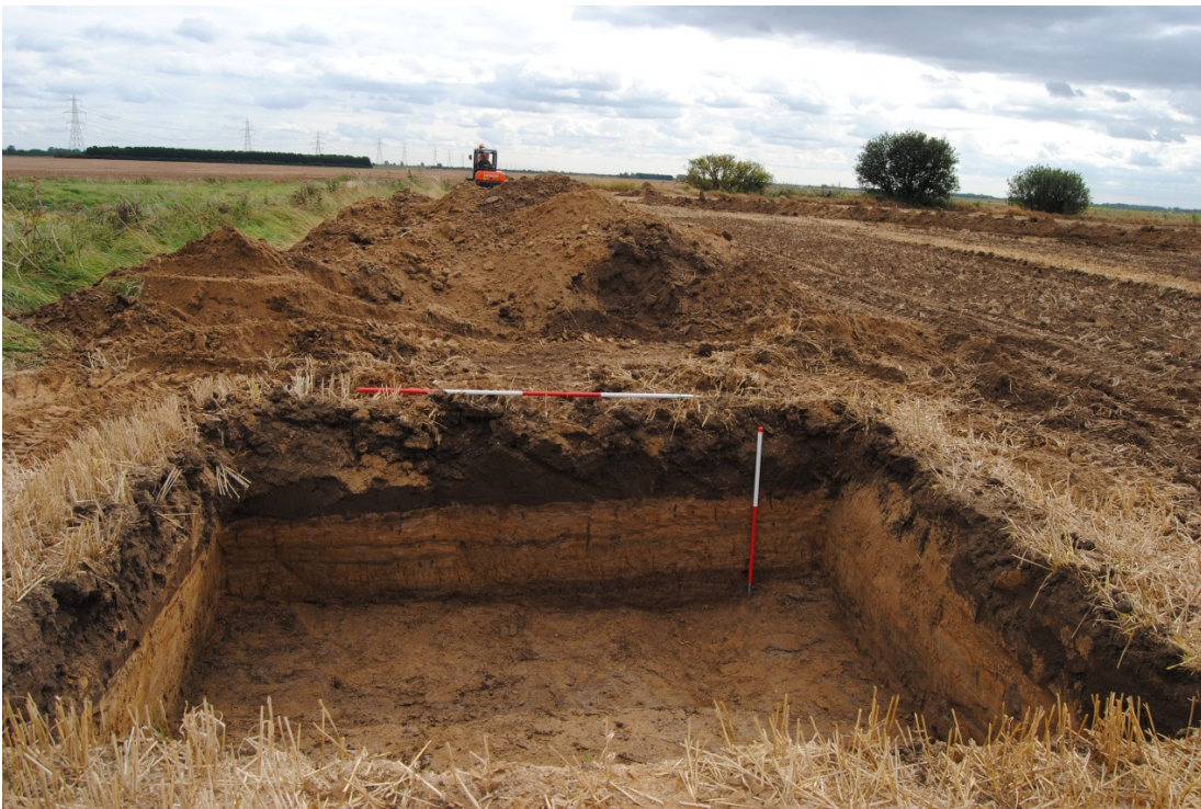
Plate 4 - Looking southeast at northwest facing section of Turbine Base B, One 1m scale, one 2m scale
