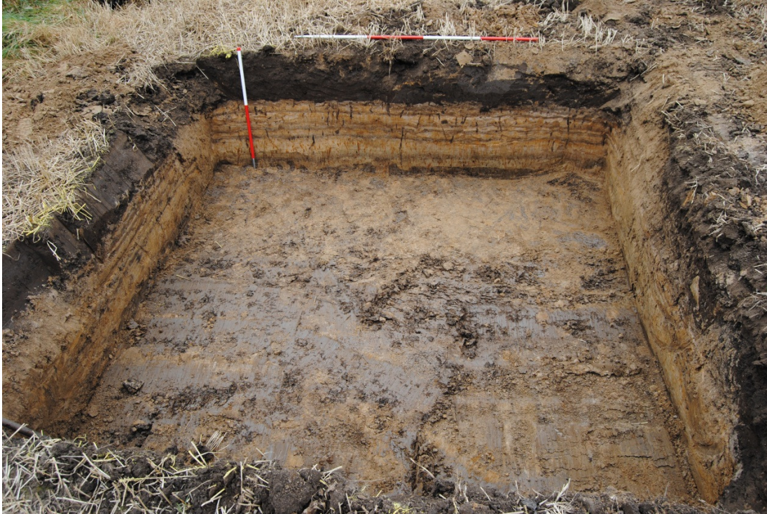
Plate 3 - Looking southwest at Turbine Base A, one 1m scale, one 2m scale
