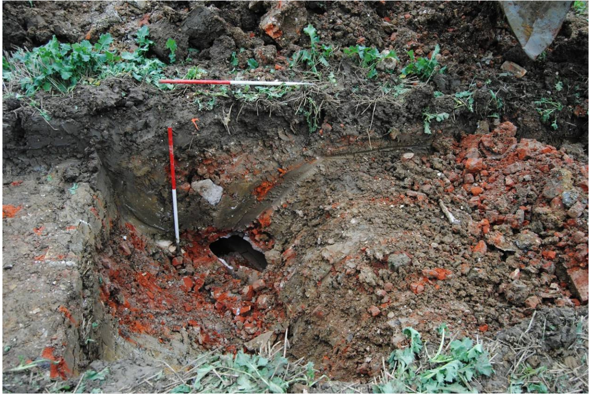
Plate 7. Looking southeast at concrete pipe in base of drain [29] (Trench 13), 1.0m scales.
