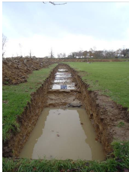
Plate 6 – Trench 4 looking southwest
