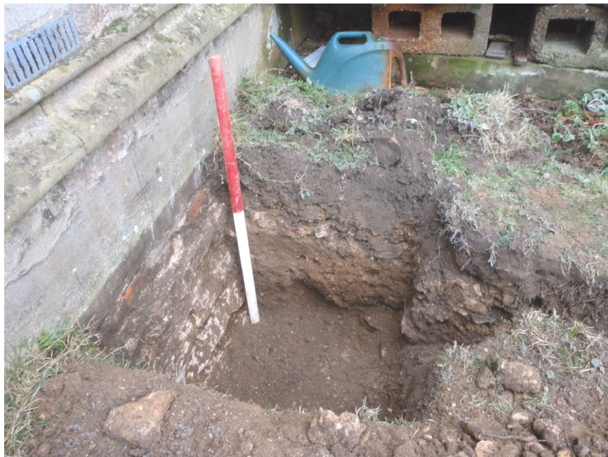
Plate 4 – Sections 5 and 6 with the rebuilt/restored north aisle (left) and associated construction deposits, looking southeast
