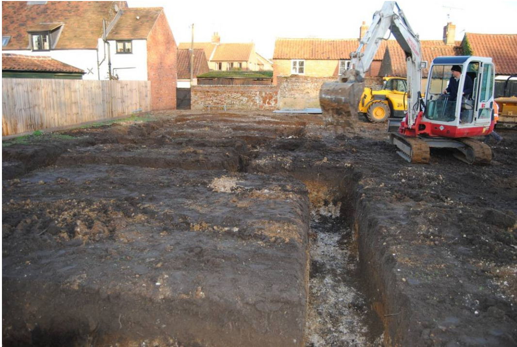
Plate 1. Looking east at excavated footing trenches.
