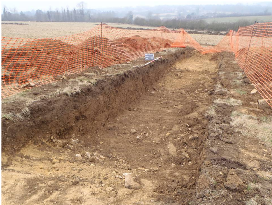
Plate 8: Section 20, feature [4044], looking SW
