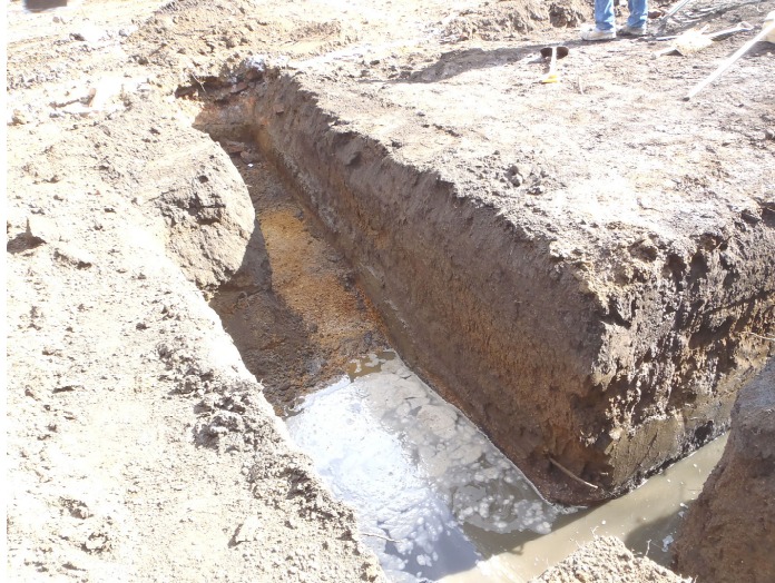
Plate 4 – Section 3 showing pond (211), looking southeast
