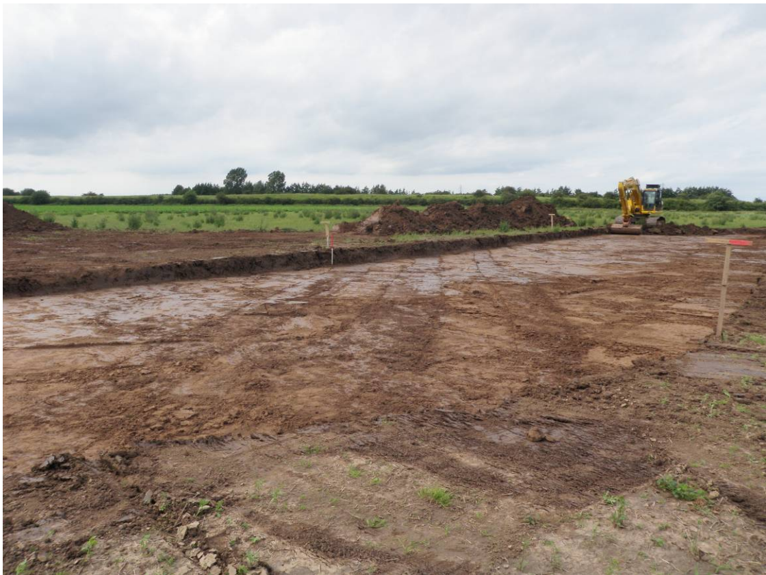
Plate 8. Road south of Turbine 6, Ditches [105], [108], [110] looking north
