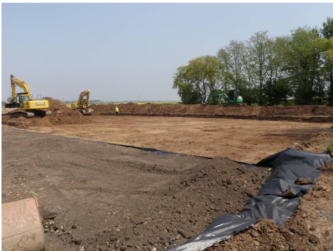
Plate 1. Machining the compound area looking northeast
