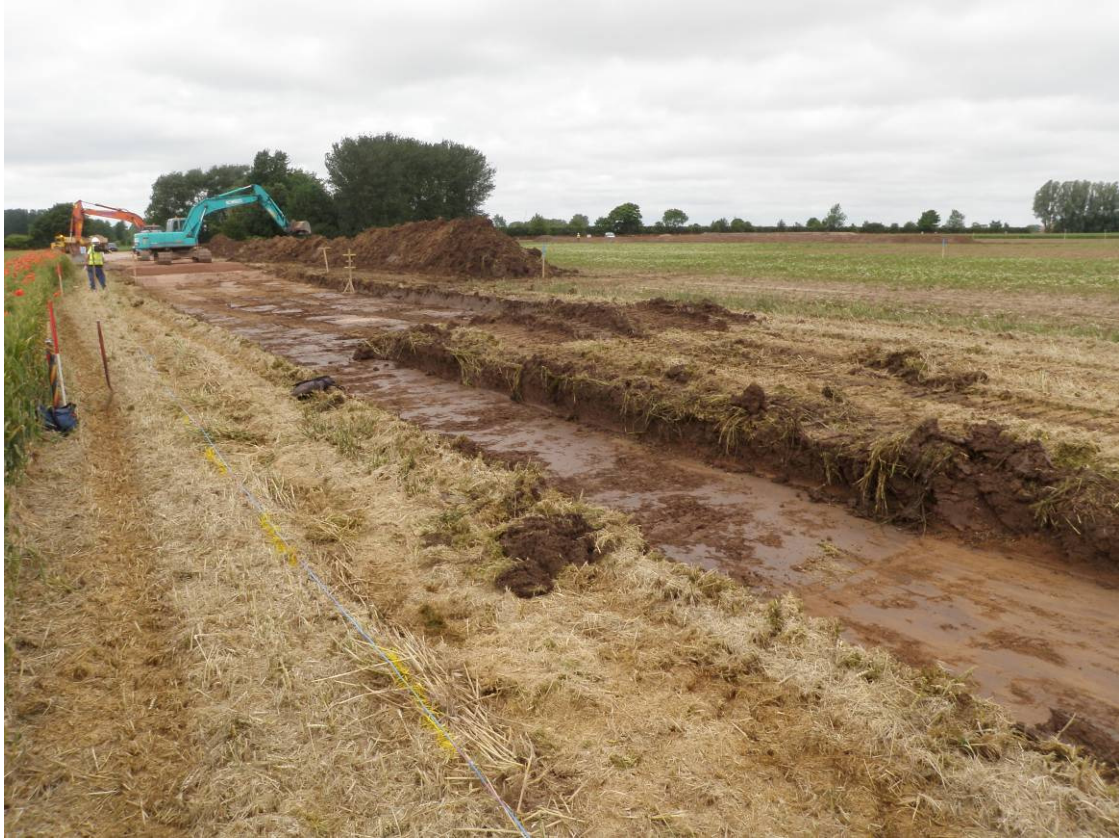
Plate 3. Road west of Turbine 2, silt (062) looking northwest
