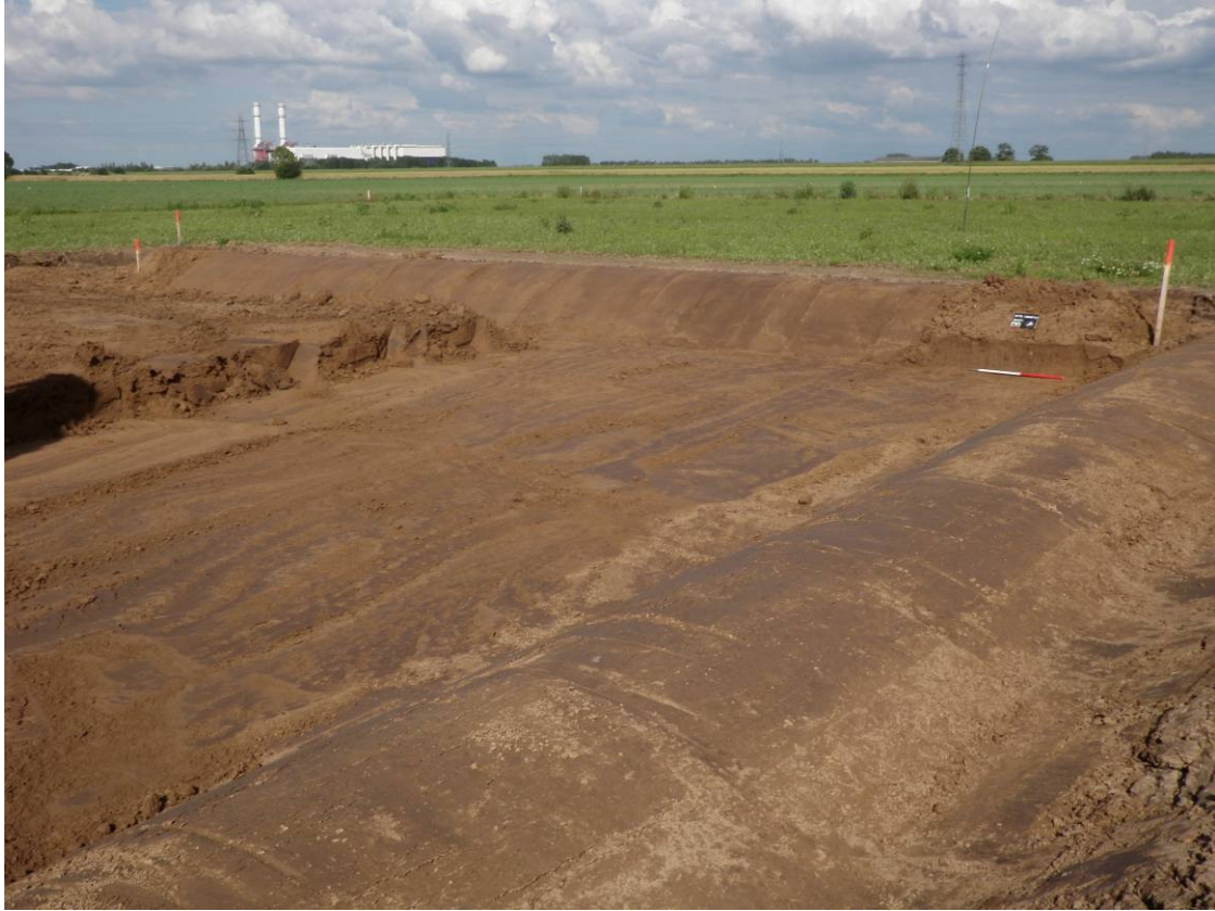
Plate 5. Turbine 4 drainage basin, channel silts (094), (095), Section 24, looking east
