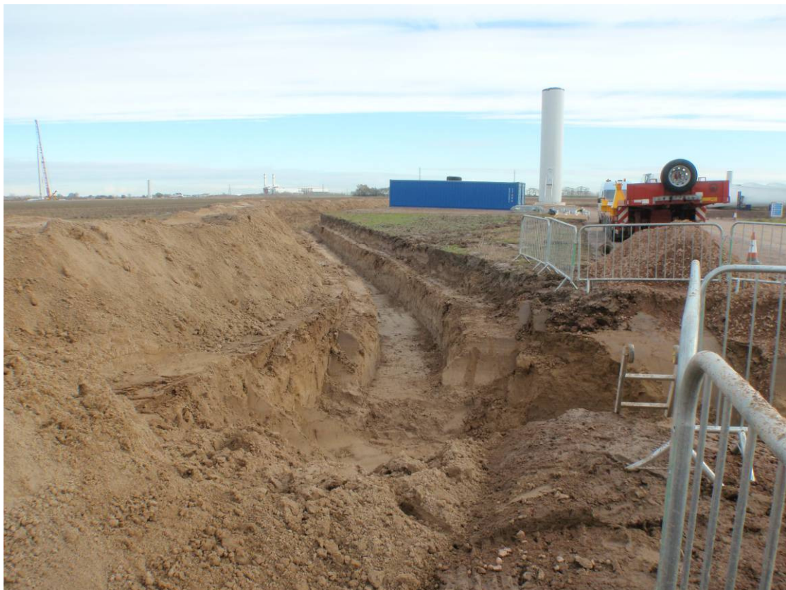
Plate 10. Cable trench at Turbine 1, looking east
