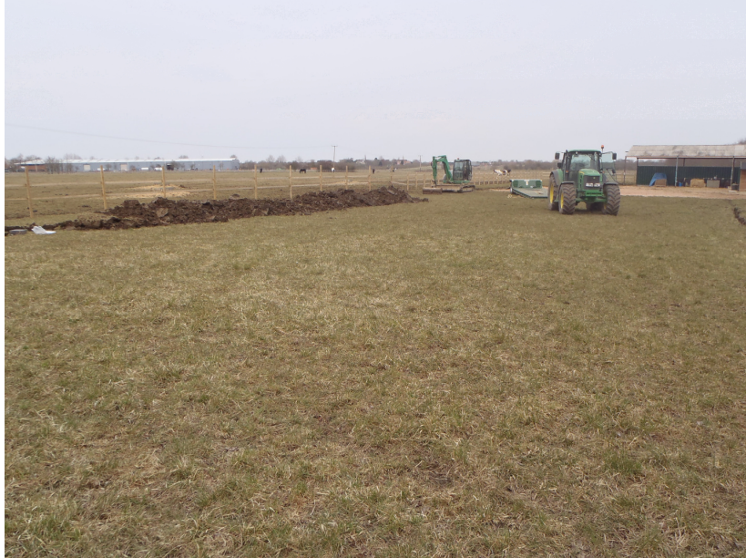
Plate 1: General shot looking north
