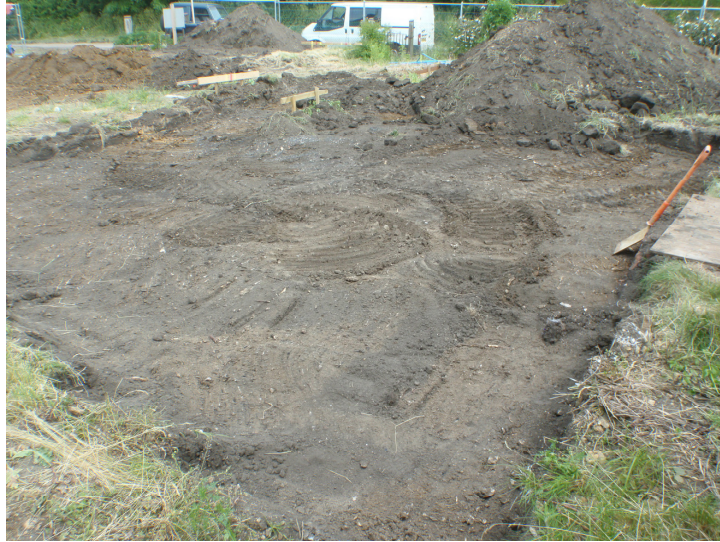
Plate 4 – The garage area after removal of overburden, looking northeast
