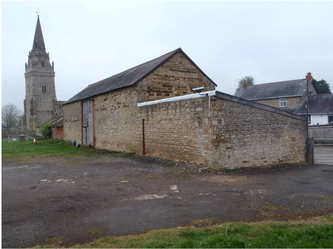
Plate 1 General site view, west side of site, looking north
