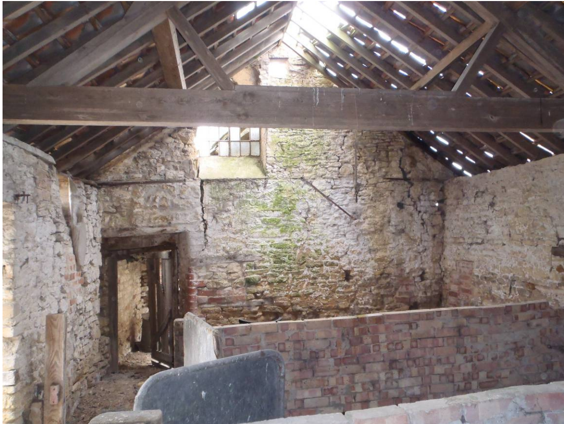
Plate 29 Building 9, western room, looking northwest
