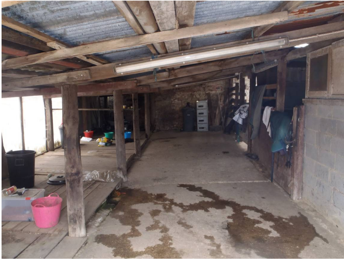
Plate 5 Building 1, northern part of building, looking east
