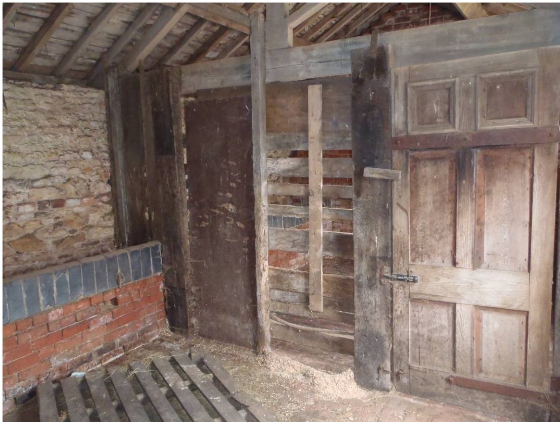
Plate 12 Building 3, western compartment, looking northeast
