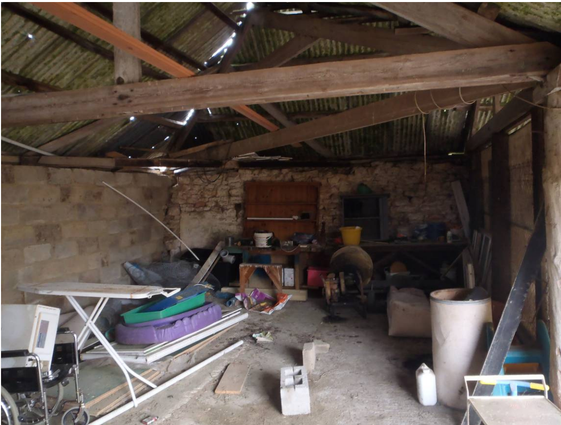
Plate 24 Building 7, northwestern room, looking north
