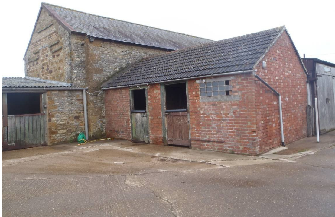
Plate 11 Building 3, south and east sides, and Building 10 to rear, looking northwest
