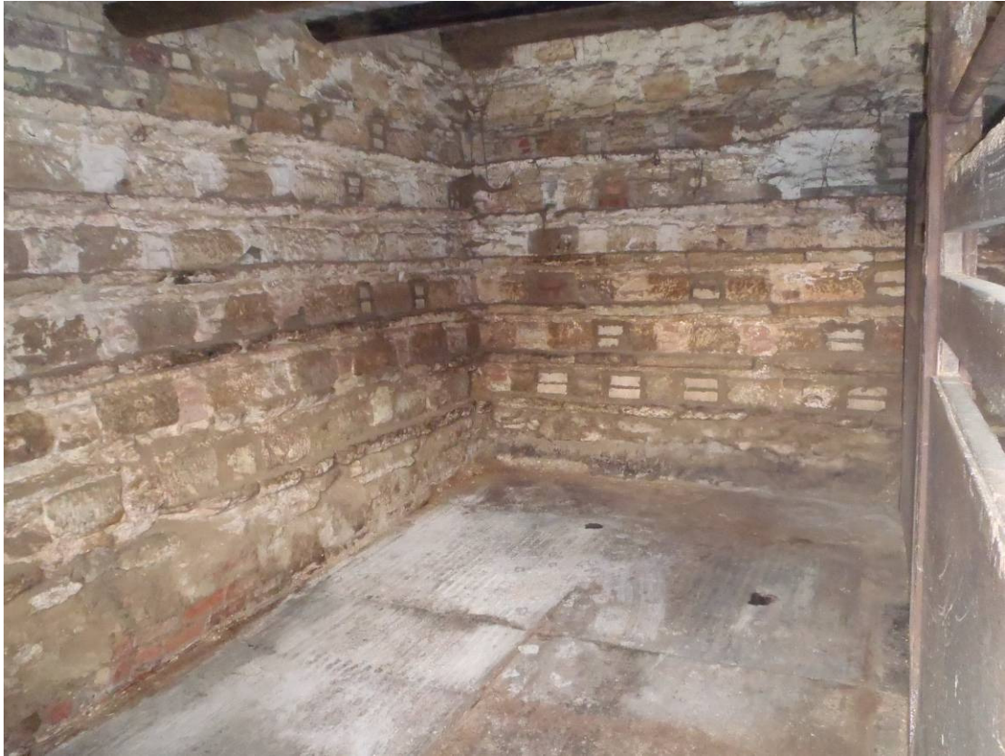
Plate 9 Building 2, southern compartment, looking southwest
