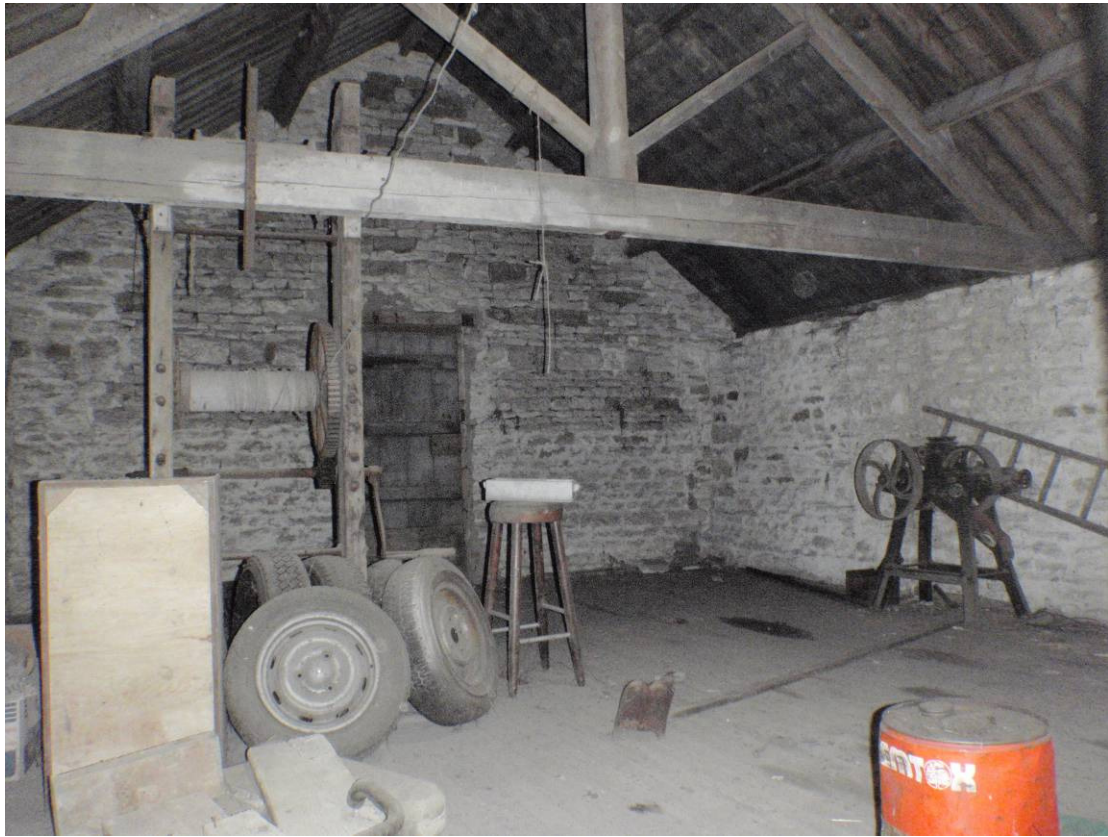
Plate 35 Building 10, upper storey, looking southwest
