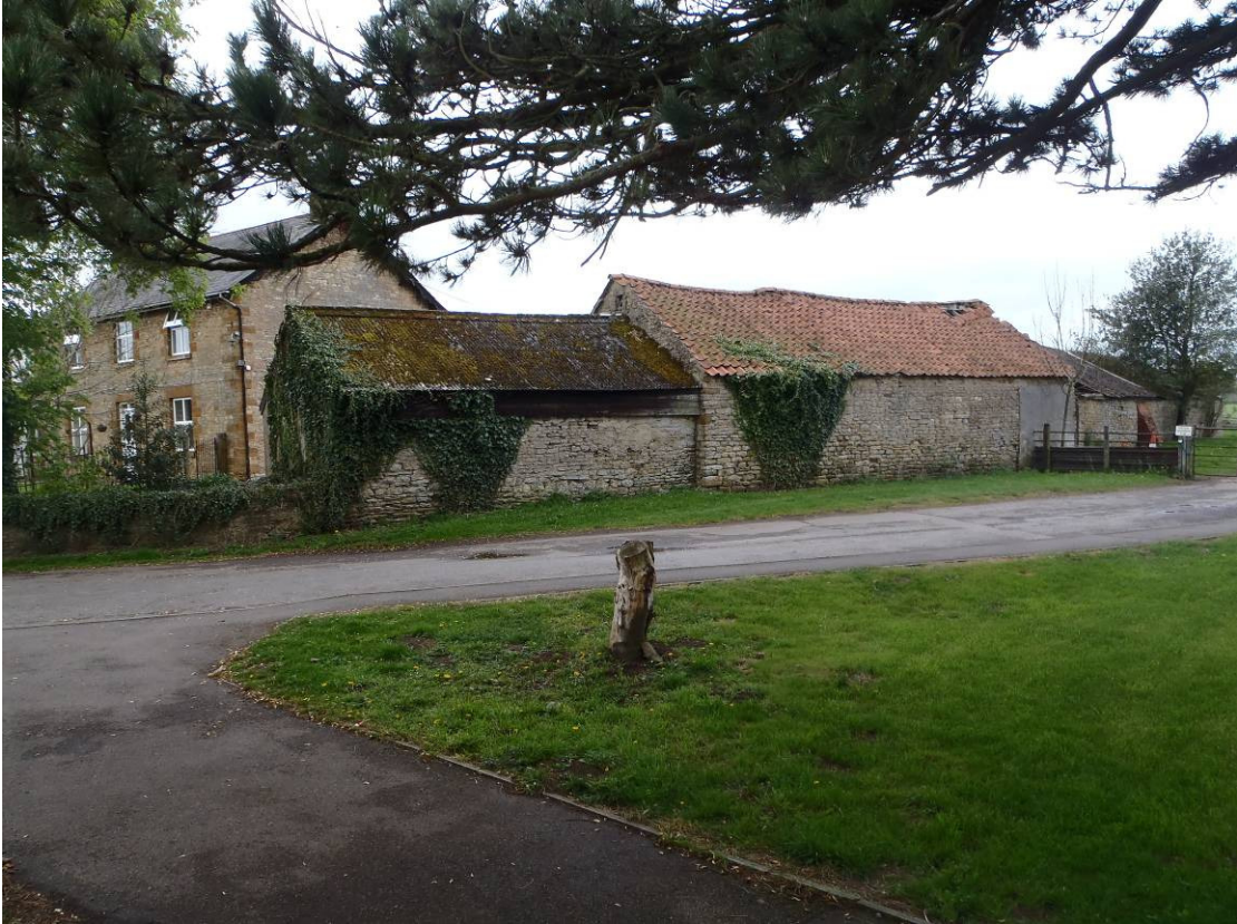
Plate 23 Rear (north side) of Buildings 7, 8 and 9, looking southwest
