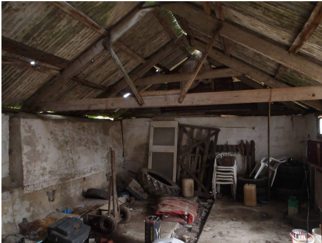
Plate 20 Building 6, looking north
