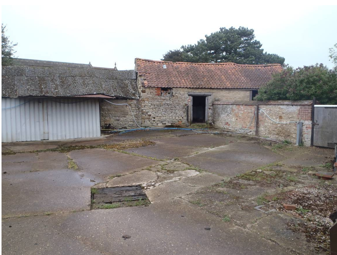
Plate 27 Building 9, southern elevation, west side, looking northeast
