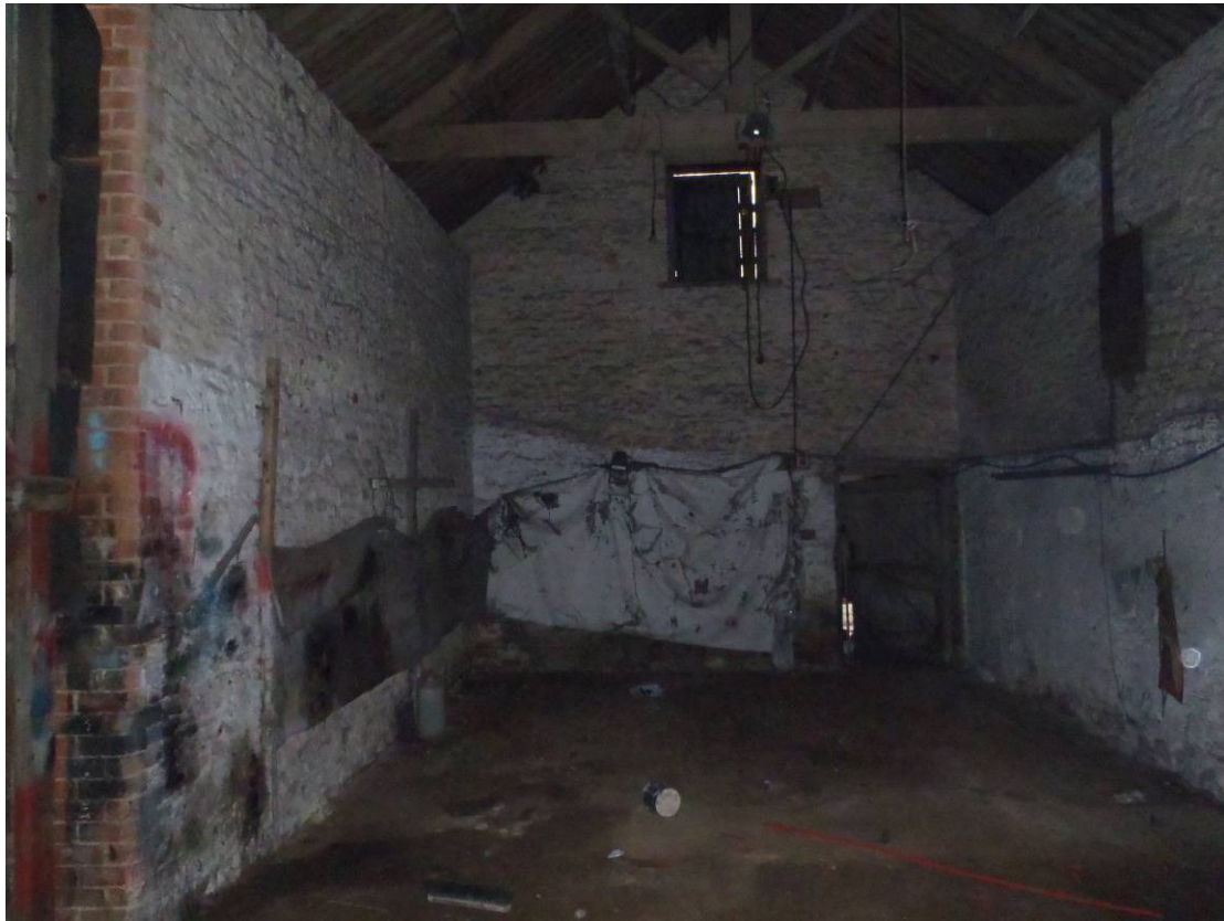
Plate 33 Building 10, looking north
