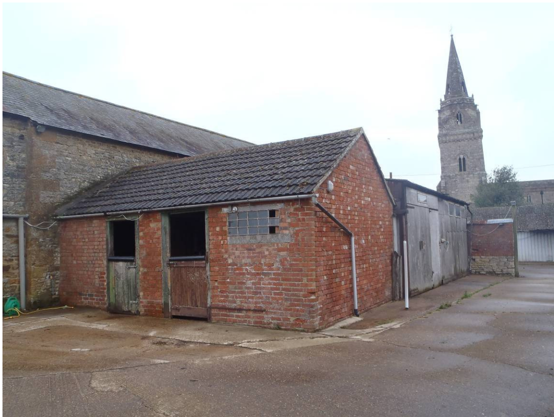
Plate 14 Building 3 and Building 4, beyond, looking north
