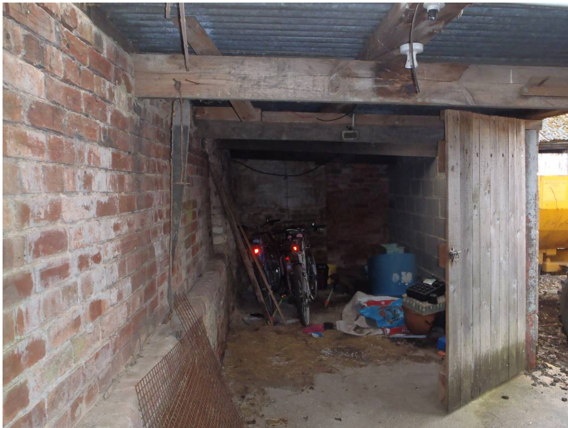
Plate 18 Building 5, interior, looking west
