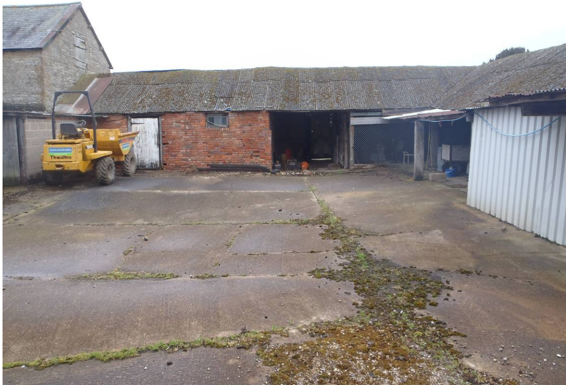
Plate 19 Buildings 6 and 7, looking west
