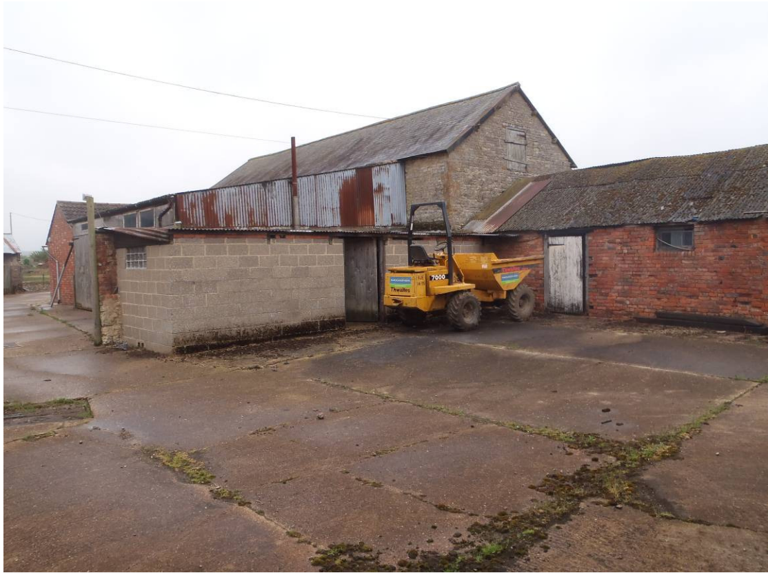
Plate 17 Building 5, north and east sides, looking southwest
