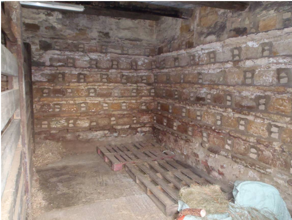
Plate 10 Building 2, northern compartment, looking west
