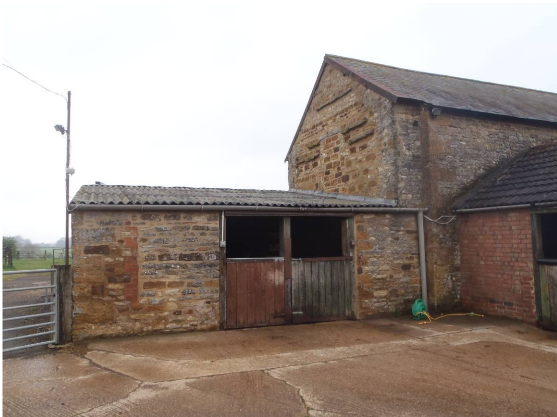
Plate 8 Building 2, eastern elevation, looking west
