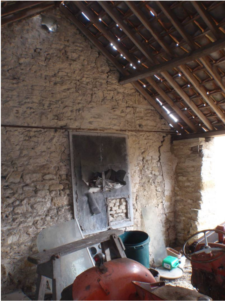
Plate 31 Building 9, eastern room, looking southeast
