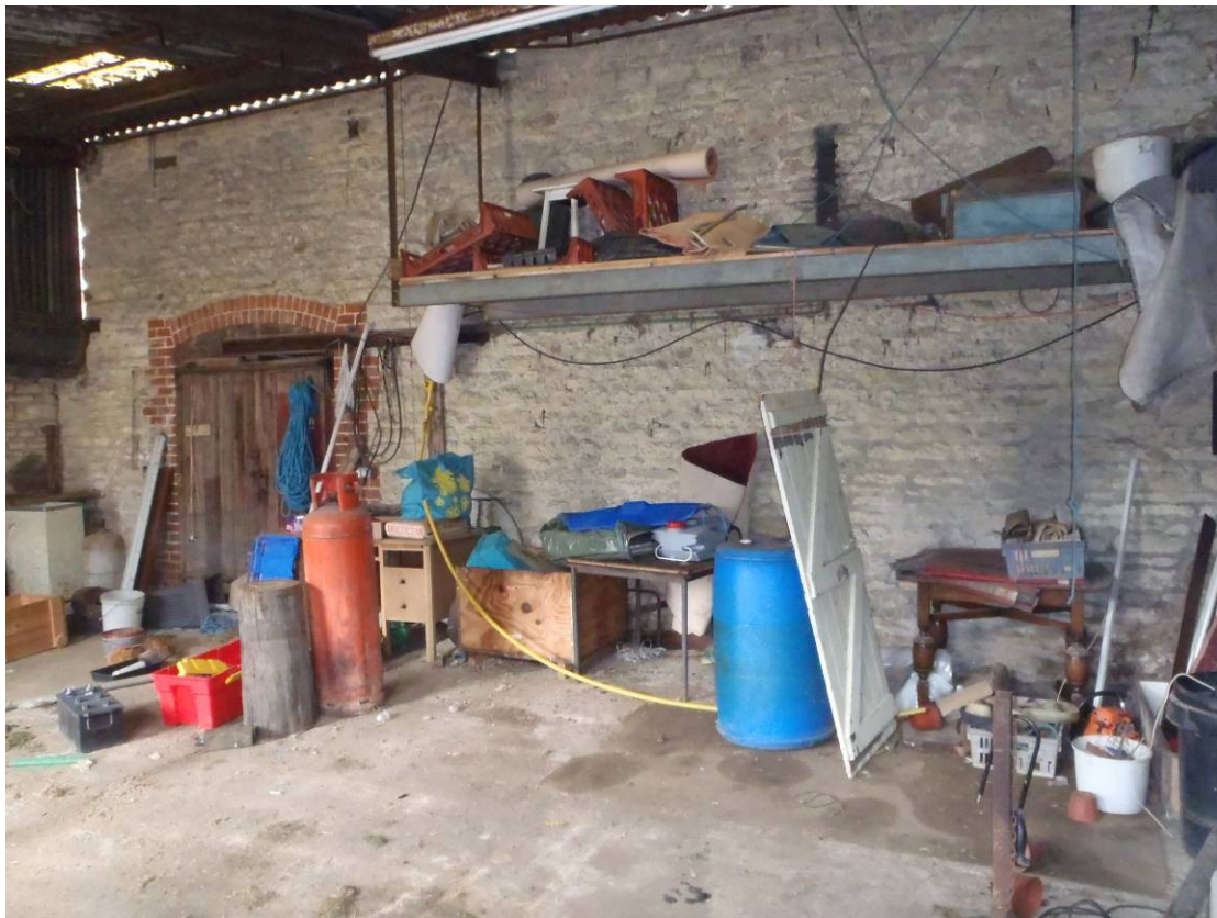
Plate 16 Building 4, western side, showing door to Building 10, looking southwest
