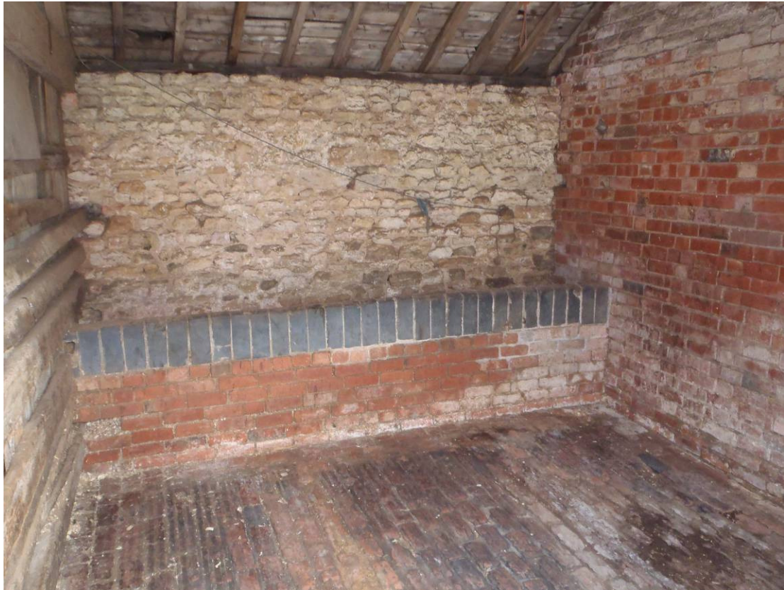
Plate 13 Building 3, eastern compartment, long north
