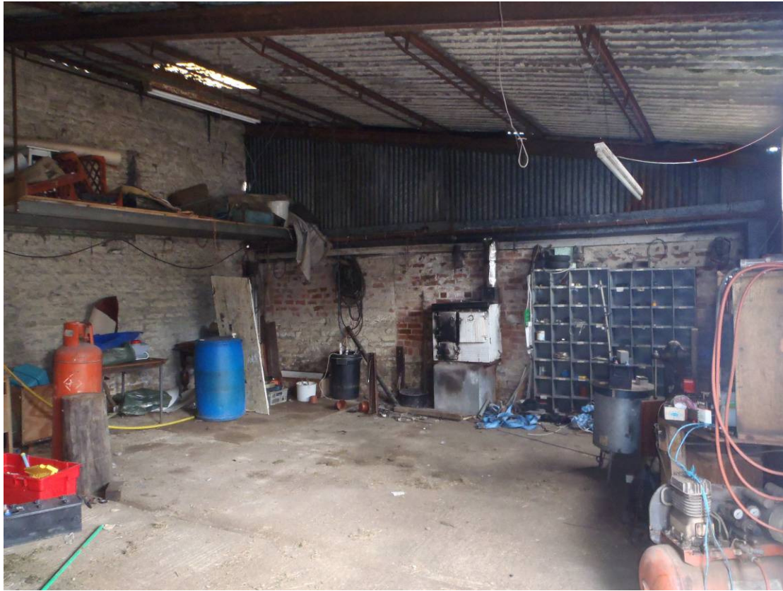
Plate 15 Building 4, interior north side, looking north
