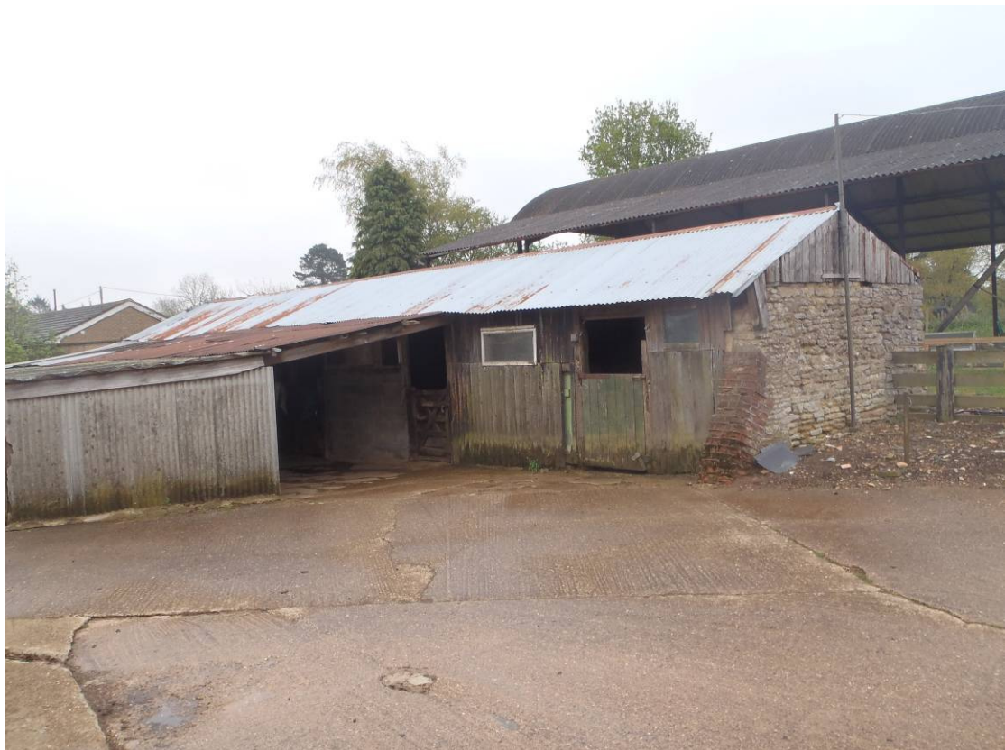
Plate 4 Building 1, north and west sides, looking southeast
