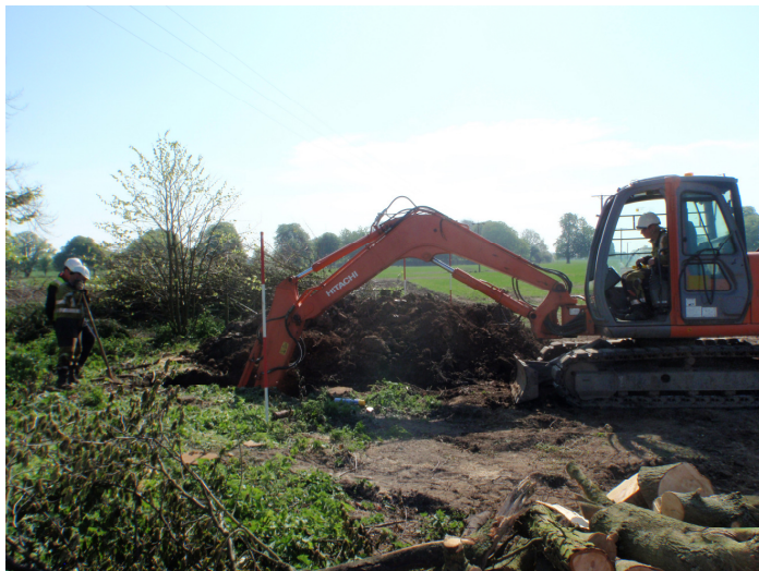
Plate 1 – Trench excavation for double pylon
