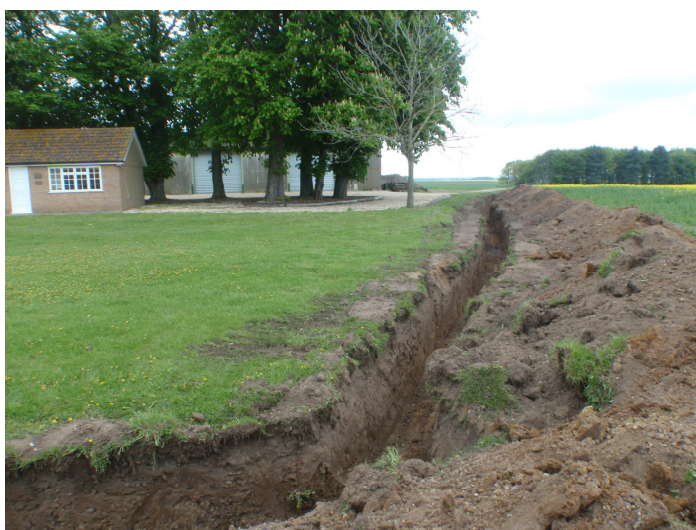
Plate 3 – Cable trench east of The Grange, looking north
