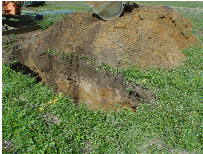
Plate 5 – Section 4, looking west
