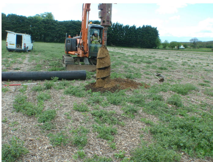
Plate 2 – Drilling borehole for single pole
