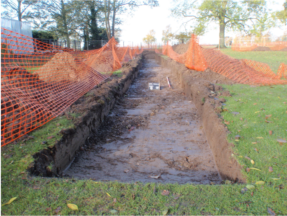
Plate 1: Trench 1 – general shot
