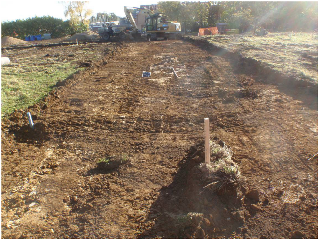
Plate 1 General Site View, looking south
