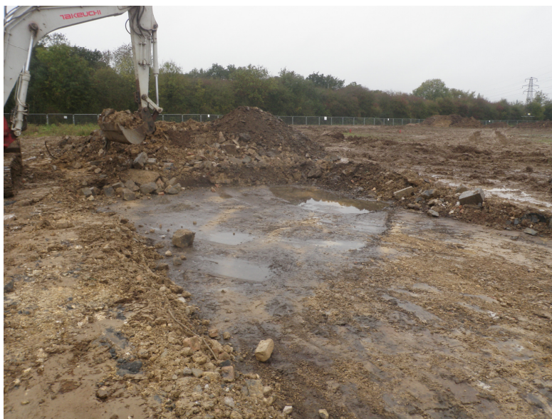
Plate 3 – The main area during initial stripping, looking northwest
