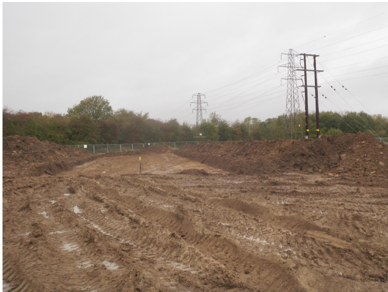
Plate 2 – The northern area following the overburden strip, looking northwest
