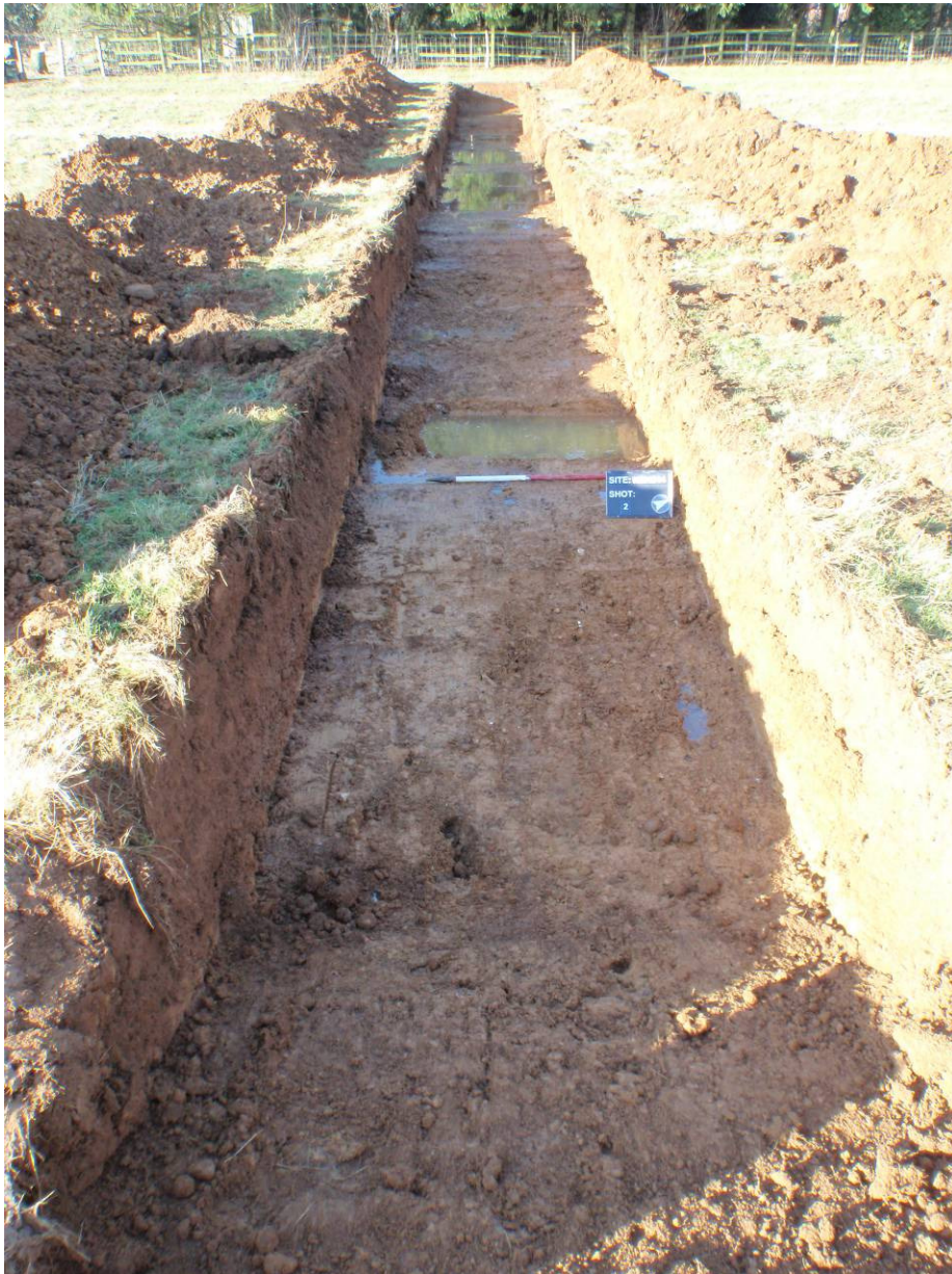
Plate 1: Trench 1, general view
