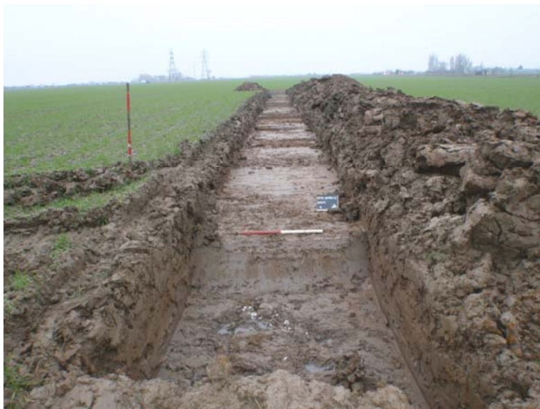
Plate 5 – Trench 3, looking southwest
