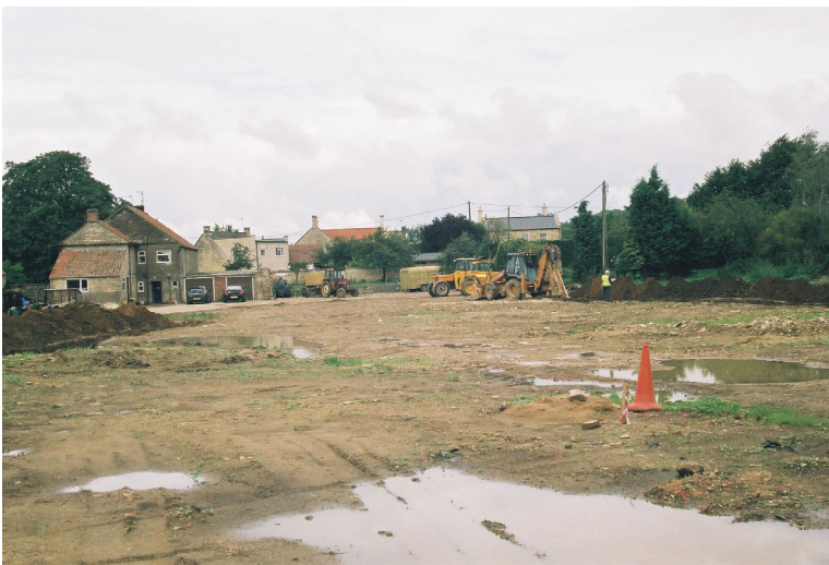
Plate 2 General view of investigation area, looking S.
