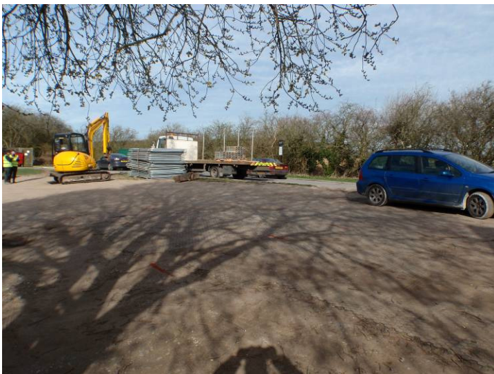
Plate 3. General view from the café showing trench locations and proximity of the roadway, looking northwest
