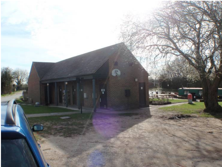
Plate 2. General view of the site showing the proximity of the café, looking approximately southeast
