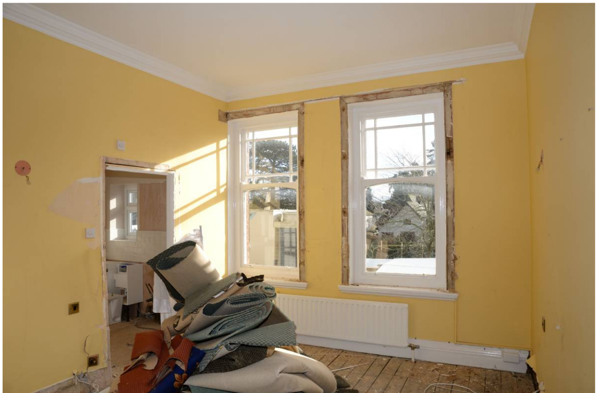
Plate 20. First floor bedroom, facing c. east
