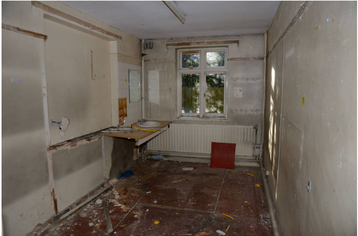
Plate 17. Room in extensions to southwest, looking southwest
