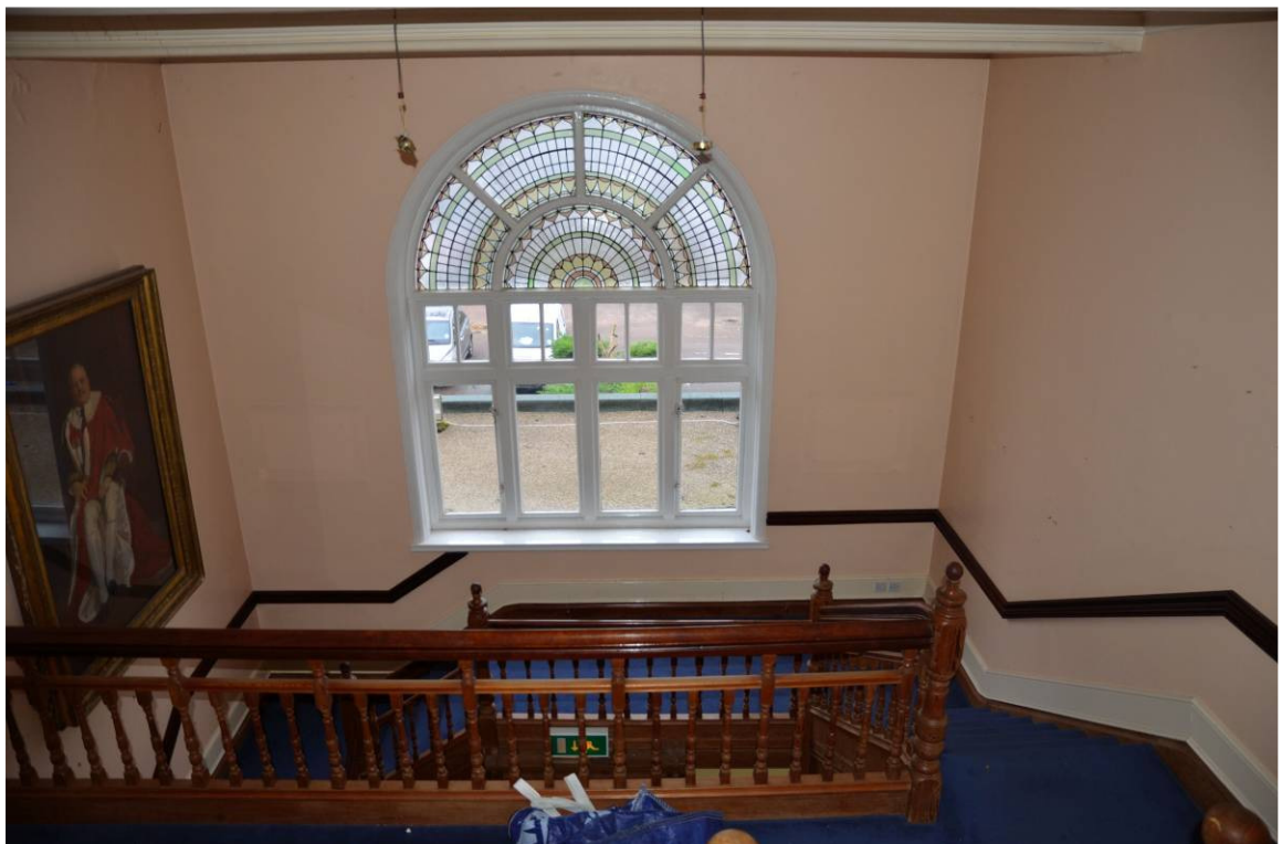
Plate 4. Interior of stairs window, looking northwest
