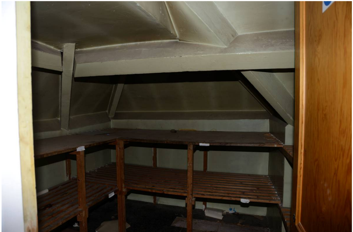
Plate 28. Storage room at second floor, northwest corner, looking west
