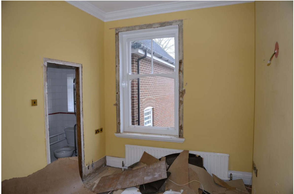
Plate 21. First floor bedroom, facing west
