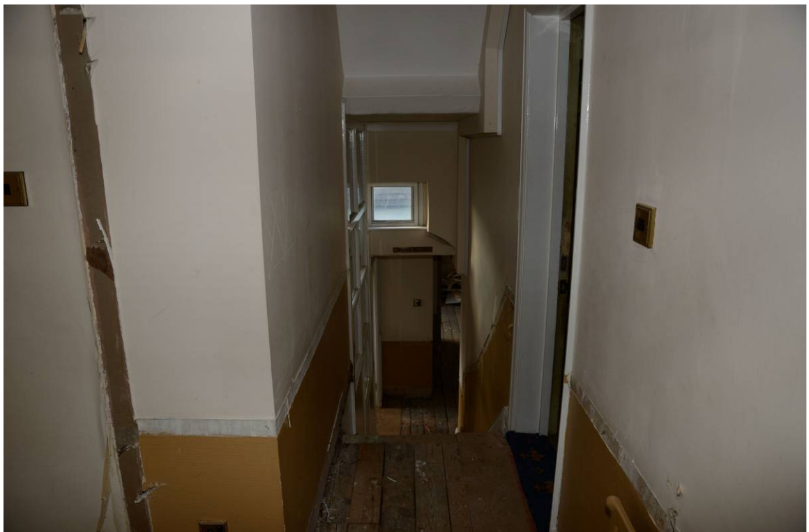
Plate 12. Second staircase from second floor, looking southwest
