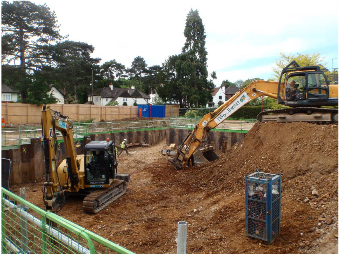
Plate 29. Machining the basement of the new building looking southwest
