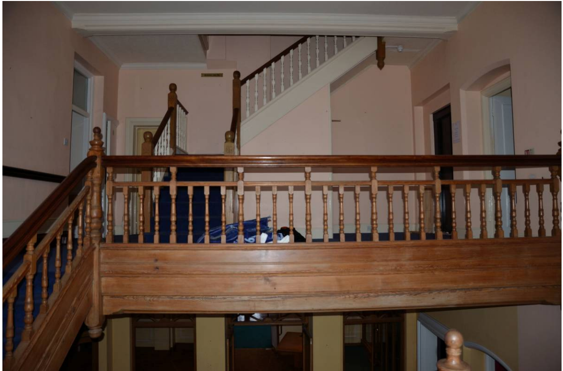
Plate 5. Landing and stairs to second floor, looking southeast
