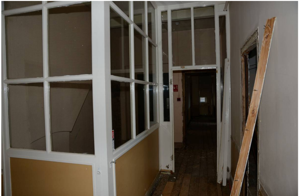
Plate 8. Second floor landing, looking southwest
