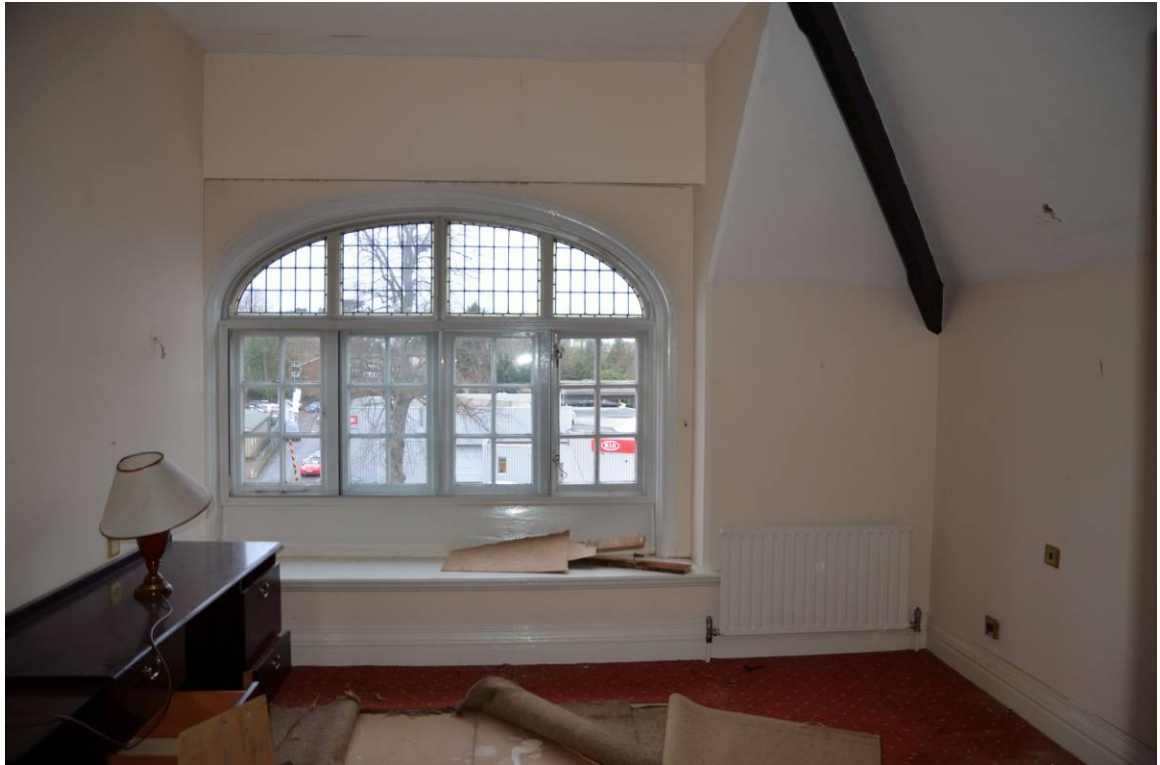
Plate 23. Second floor window in projecting bay to northwest, facing northwest
