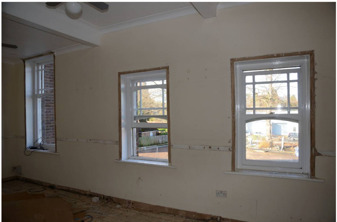
Plate 22. First floor rooms, facing west
