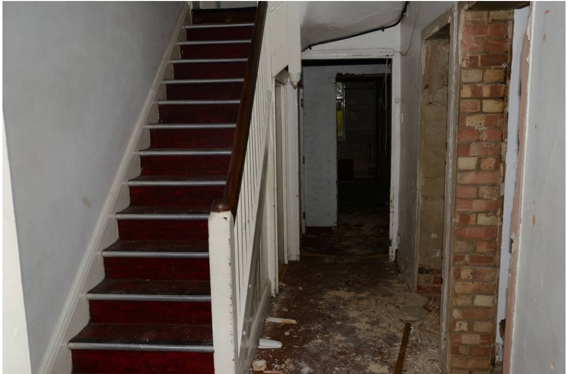
Plate 9. Original southwest door and second staircase, looking southwest
