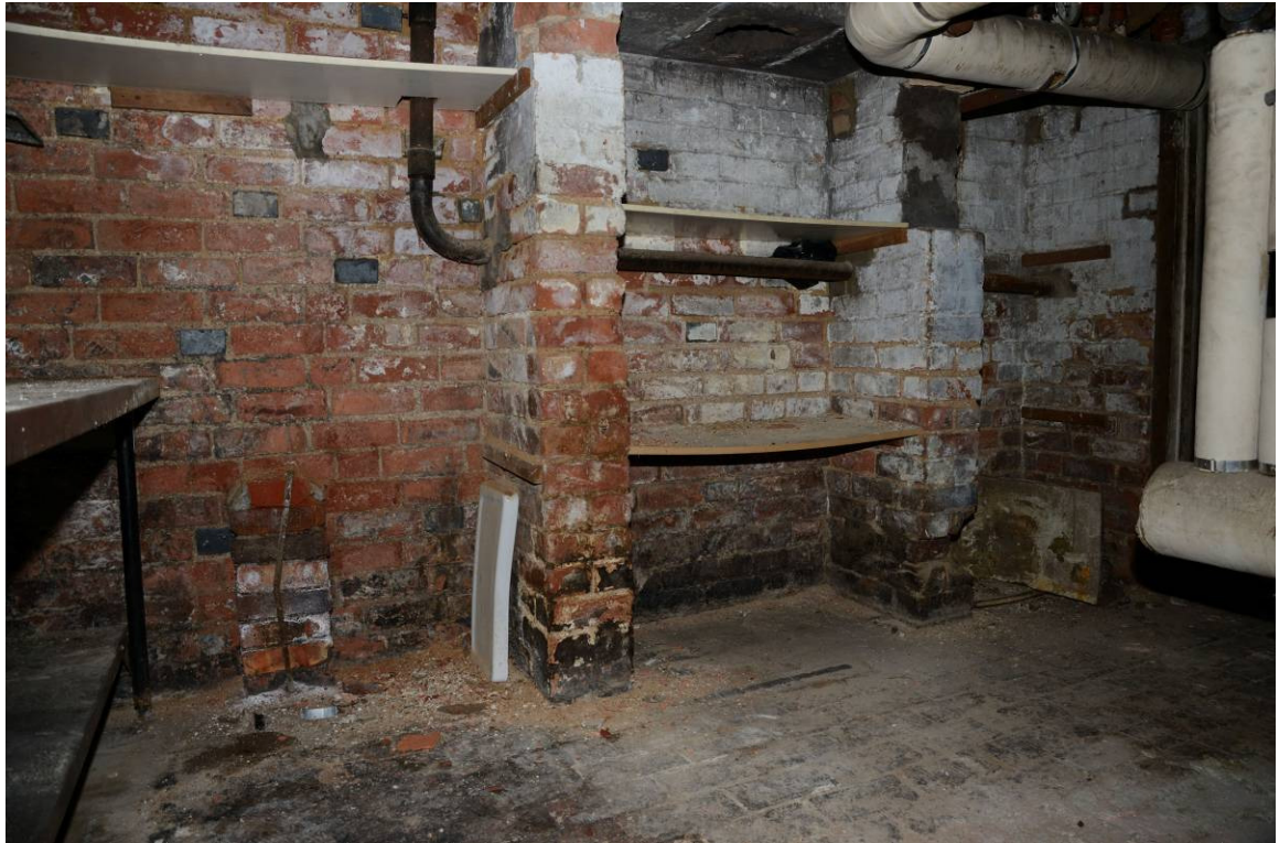
Plate 15. Basement northwest of the stairs, looking east
