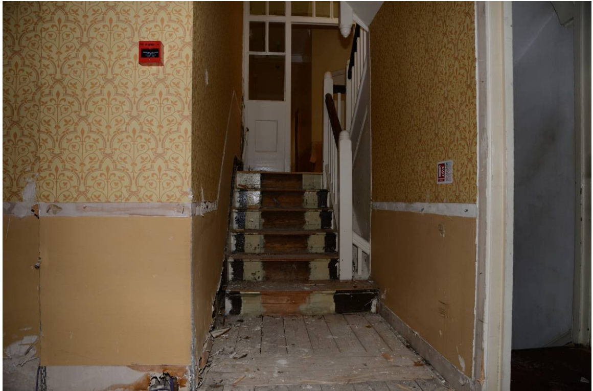
Plate 11. Second staircase from first floor, looking northeast
