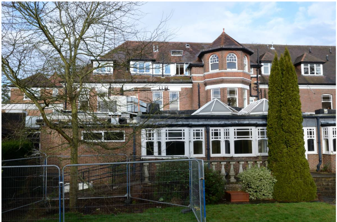
Plate 2. South facing elevation looking c. northwest
