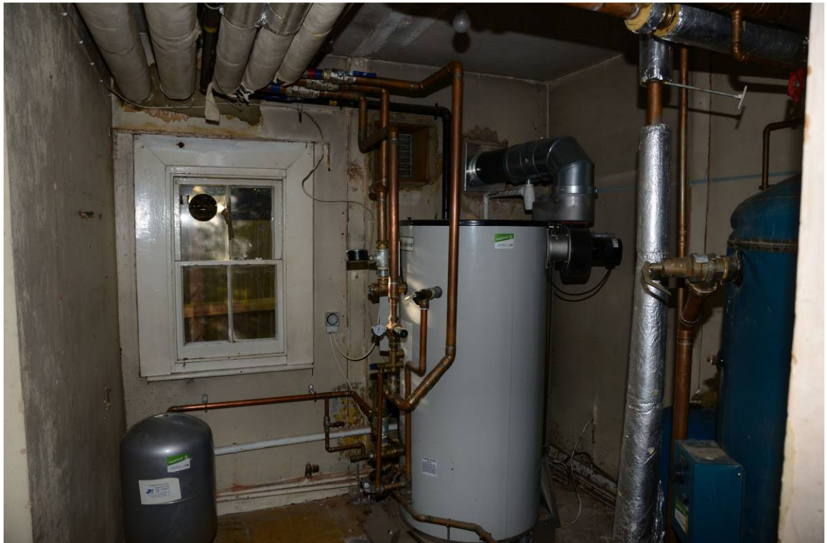
Plate 16. 'Boiler room'. looking c. west
