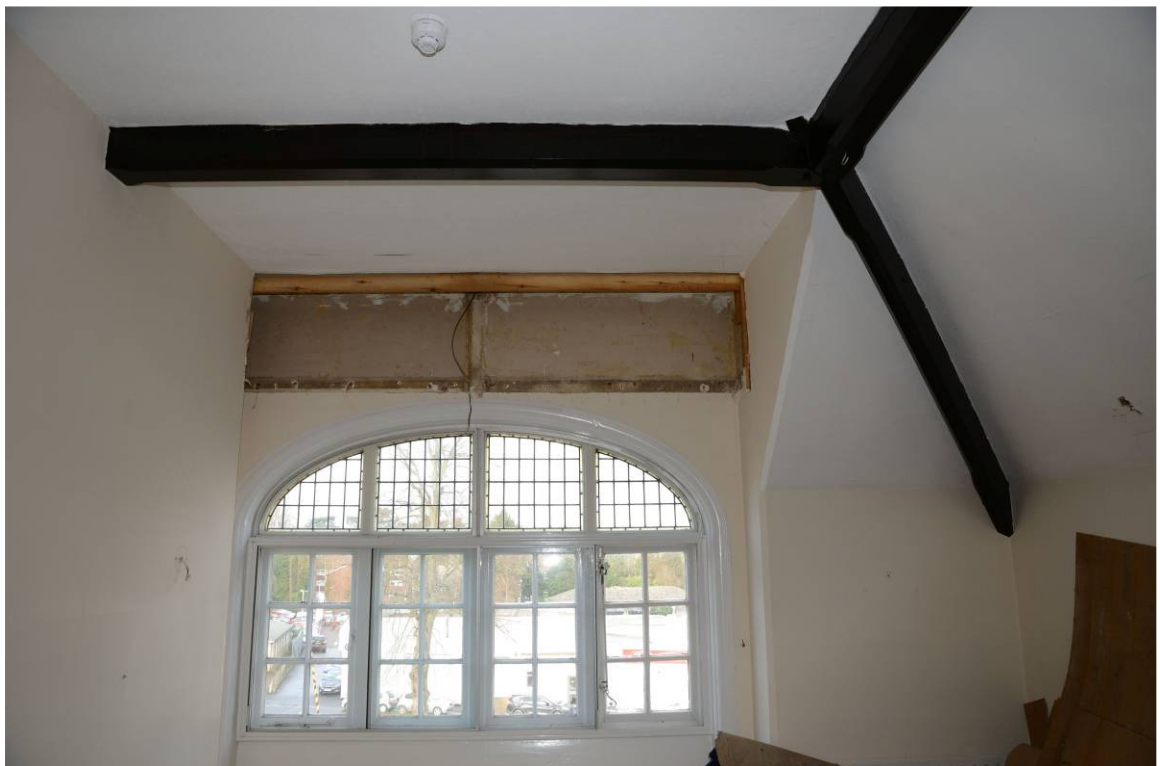
Plate 24. Exposed roof timbers in the projecting bay, facing northwest
