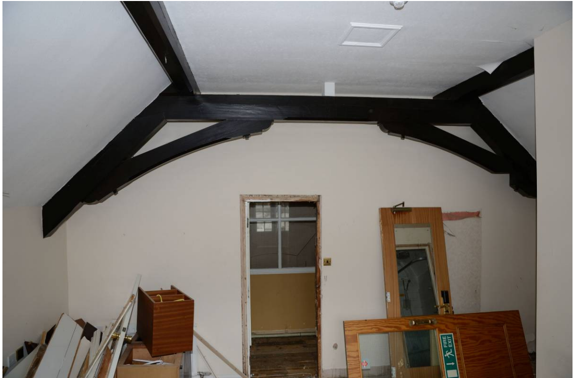
Plate 25. Exposed roof timbers in the projecting bay, facing southeast
