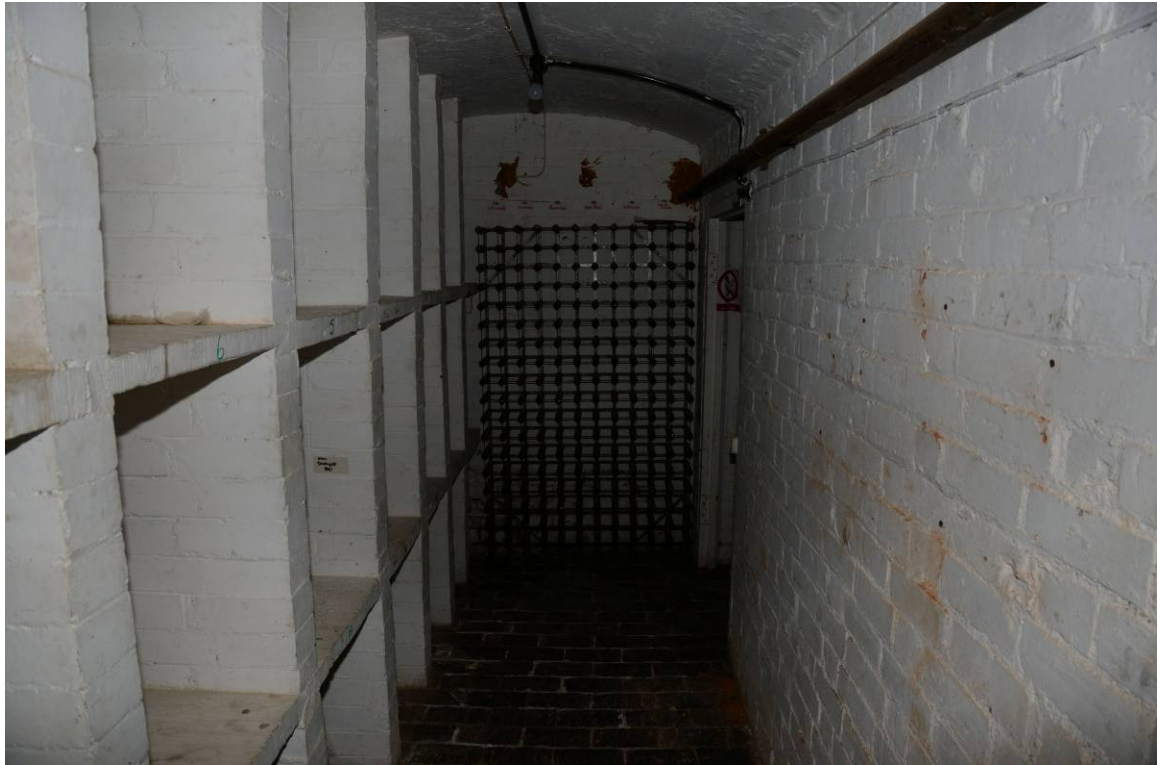
Plate 13. Basement storage area, looking northwest
