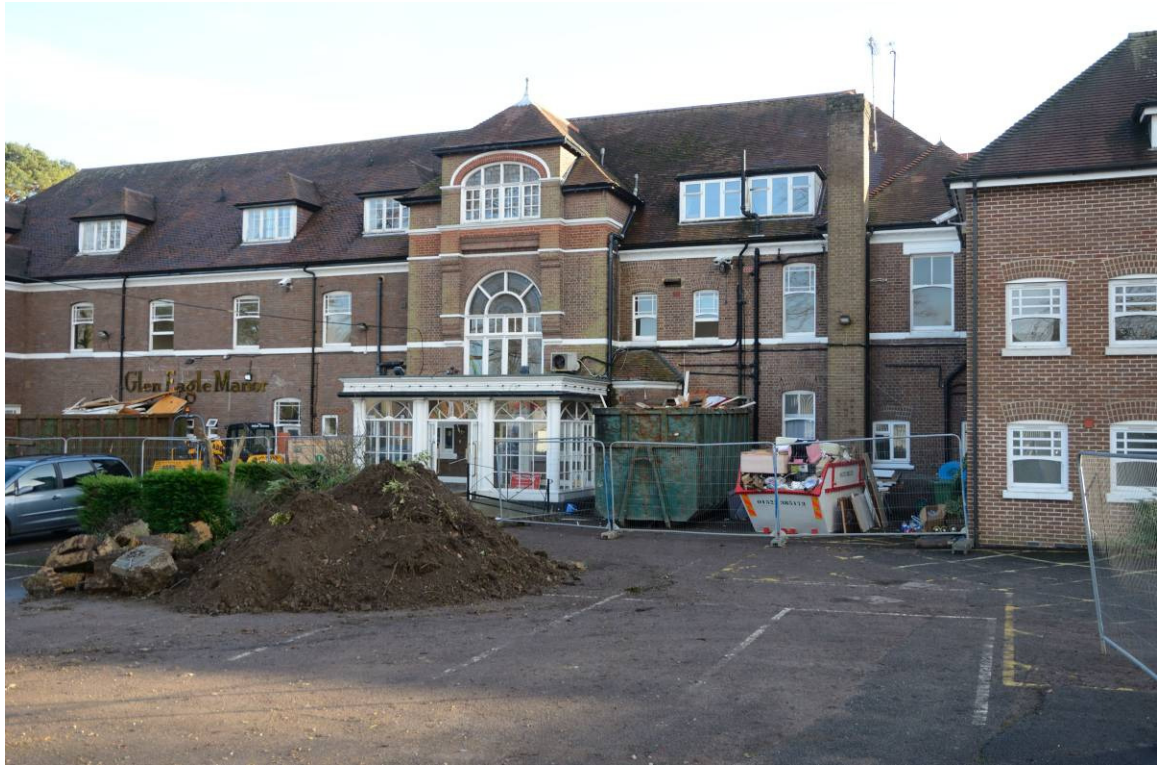
Plate 1. North facing elevation, looking c. southeast
