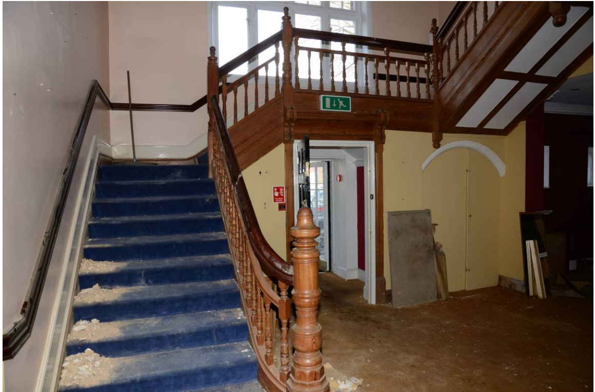
Plate 3. Staircase viewed from ground floor level facing NNW
