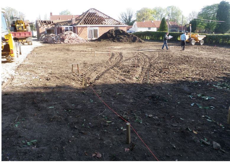
Plate 1 – View looking north across the development area
