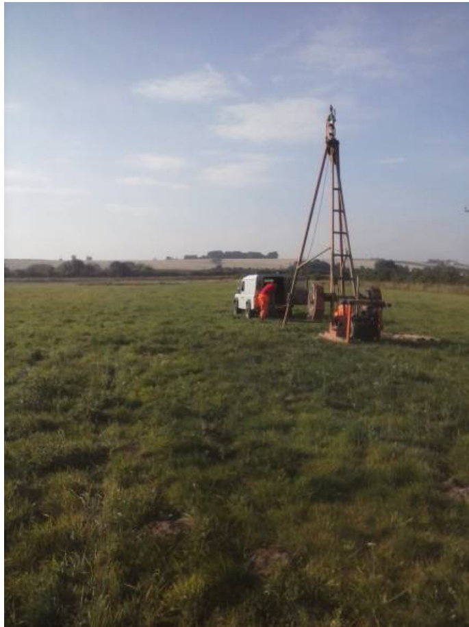
Plate 1 - General view of site and borehole equipment (BH 716)
