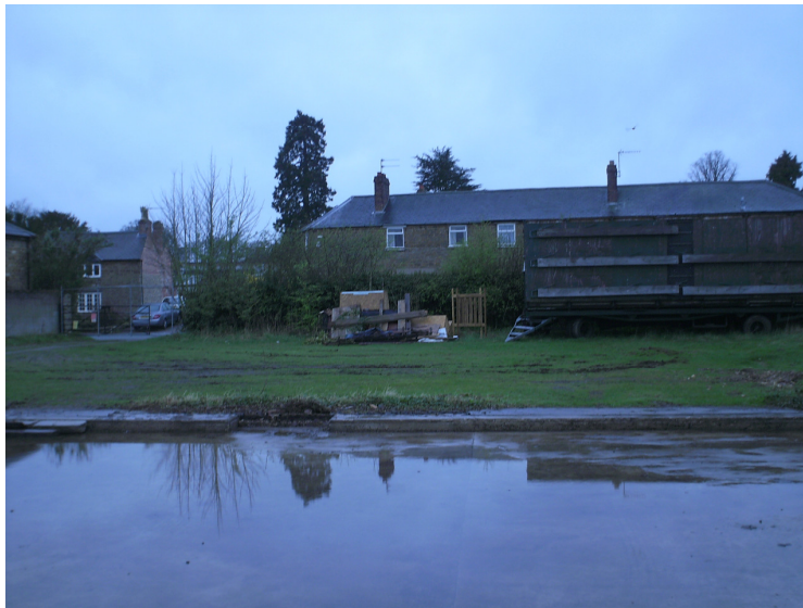
Plate 2. Location of Trench 2 prior to excavation from the concrete building pad in the centre of the site. On the left of the picture is the access from Main Road. Looking WSW.
