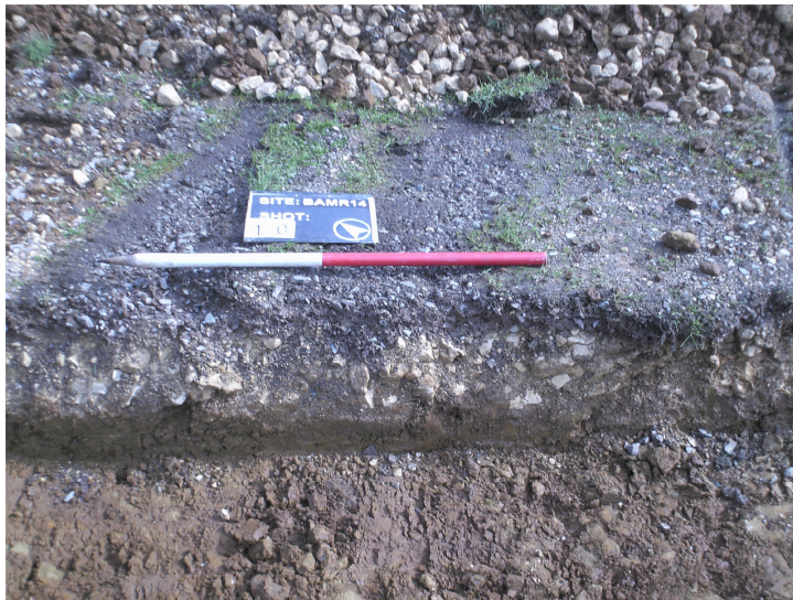
Plate 9. Representative section for Trench 2 showing the limestone hardcore and tarmac hardstanding over the remains of the subsoil. Looking northeast.
