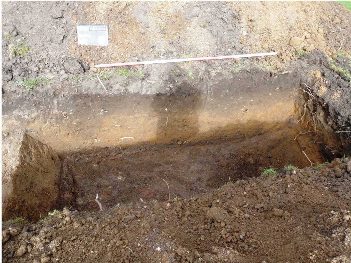
Plate 7: Trench 3, Section 6, showing made ground deposits overlying the silty backfill (308) of Car Dyke (following second phase of machining)
