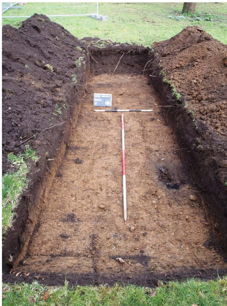
Plate 6: Trench 3, general view, looking east (after initial machining)
