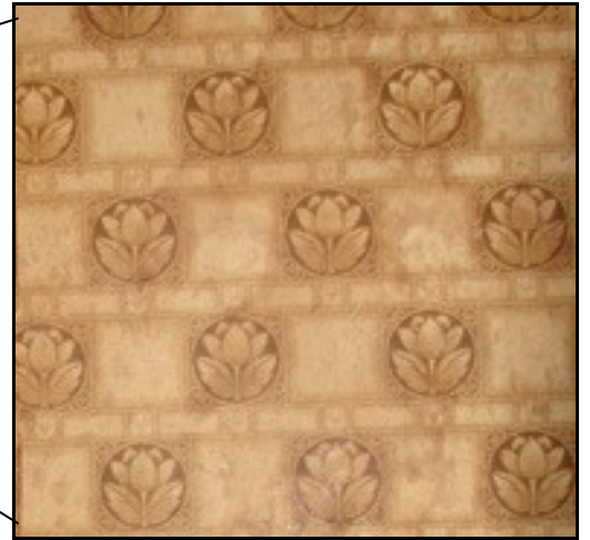
Plate 20. View of first floor north staircase illustrating possible 1930s wallpaper enlarged above
