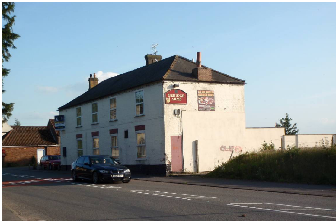
Plate 10: View of pub building (Building 2), looking southwest
