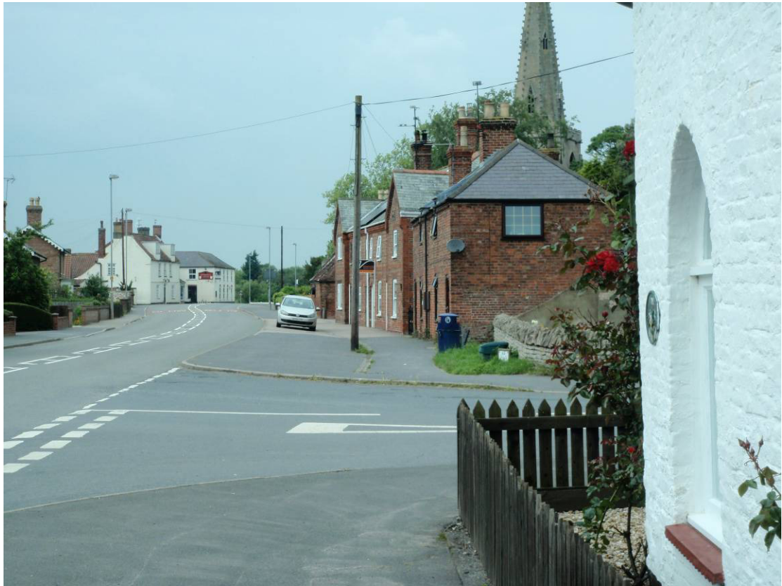
Plate 7 View from Roundhouse/Lodge Listed Building toward Site, looking northwest
