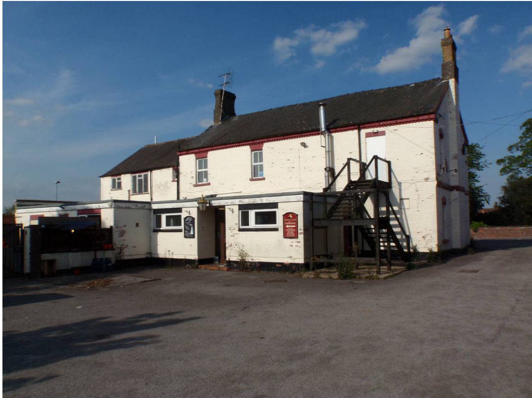
Plate 7: South and west elevation of Building 1, looking northeast, with modern single storey addition, and Building 3 abutting to the north
