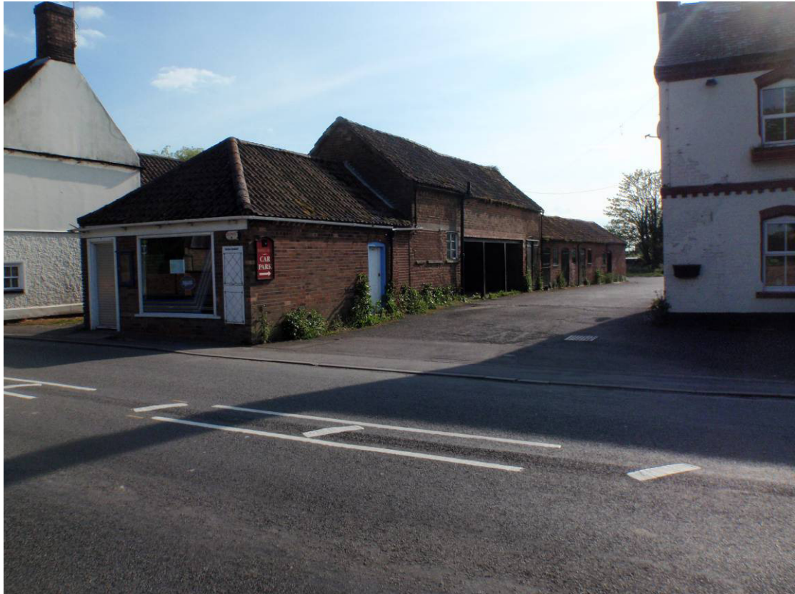
Plate 3: Block 2 outbuildings, looking southwest
