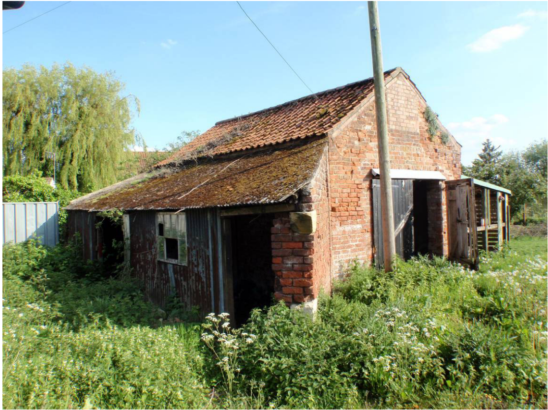
Plate 22: Extension to northeast of Building 8, looking south
