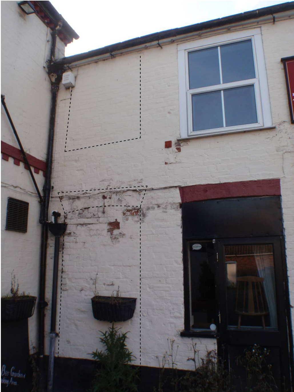
Plate 11: South elevation of Building 2, with blocked window and doorway
