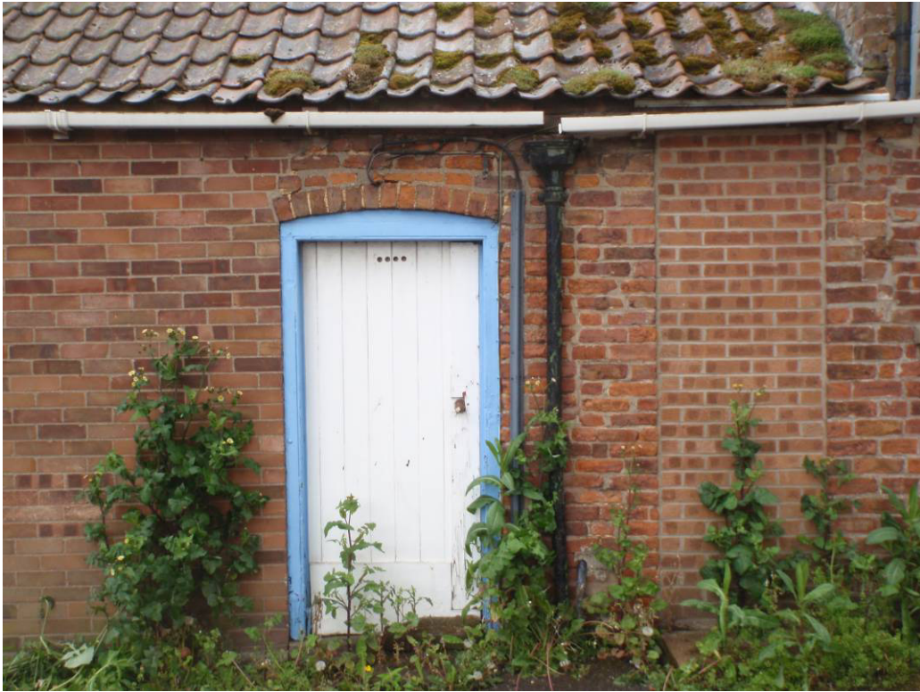
Plate 16: North side of Building 5, looking south
