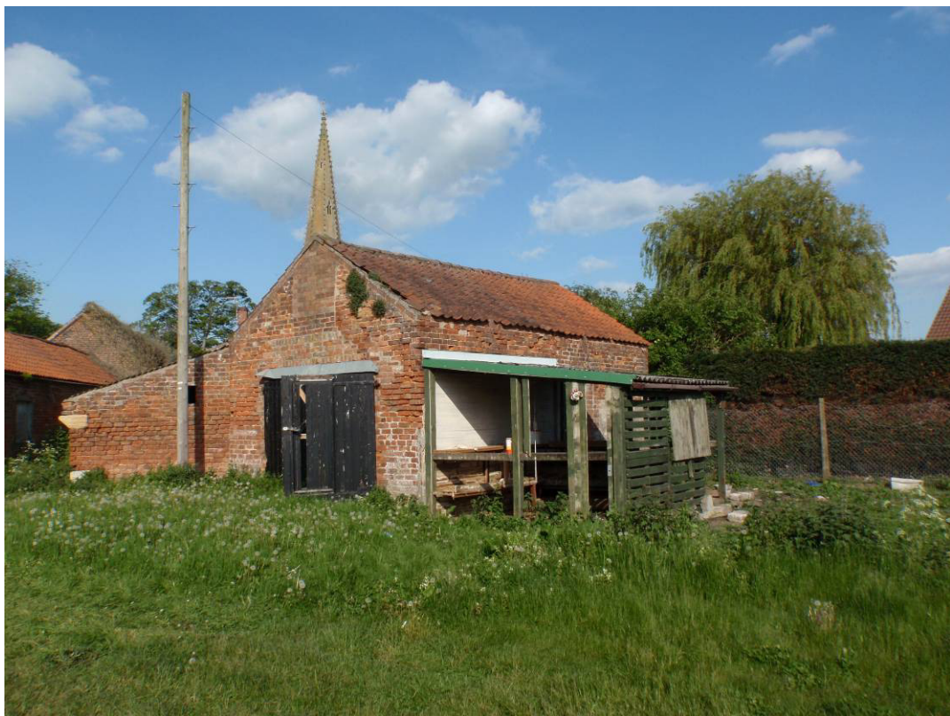
Plate 4: The small outbuilding and extensions referenced as Block 3, looking east
