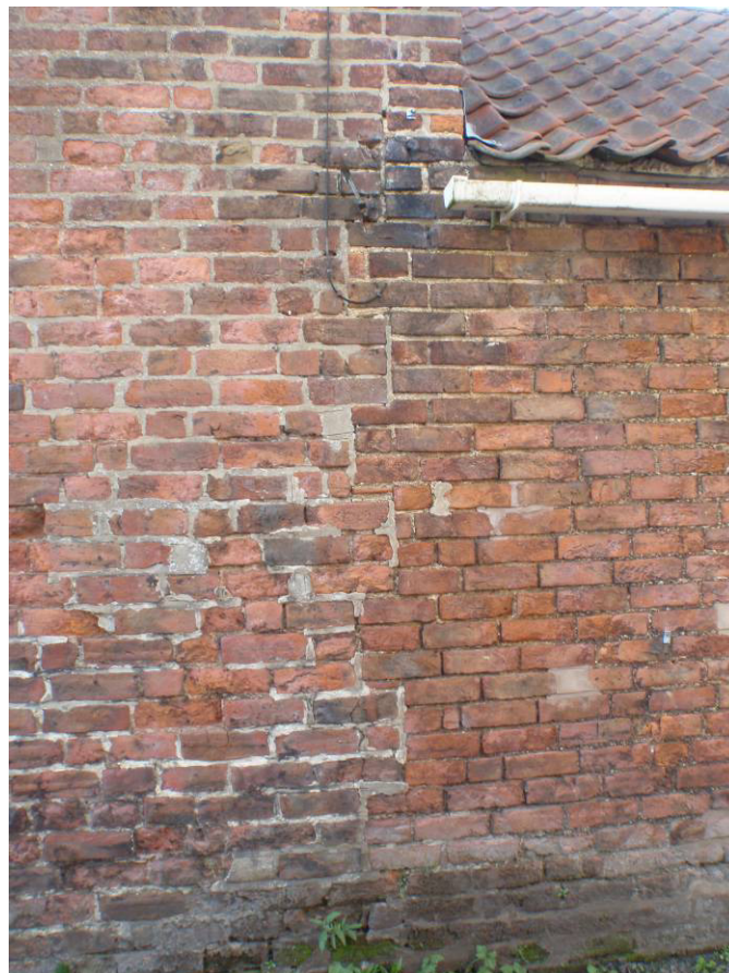
Plate 15: South side of Building 5 at the keyed joint with Building 6
