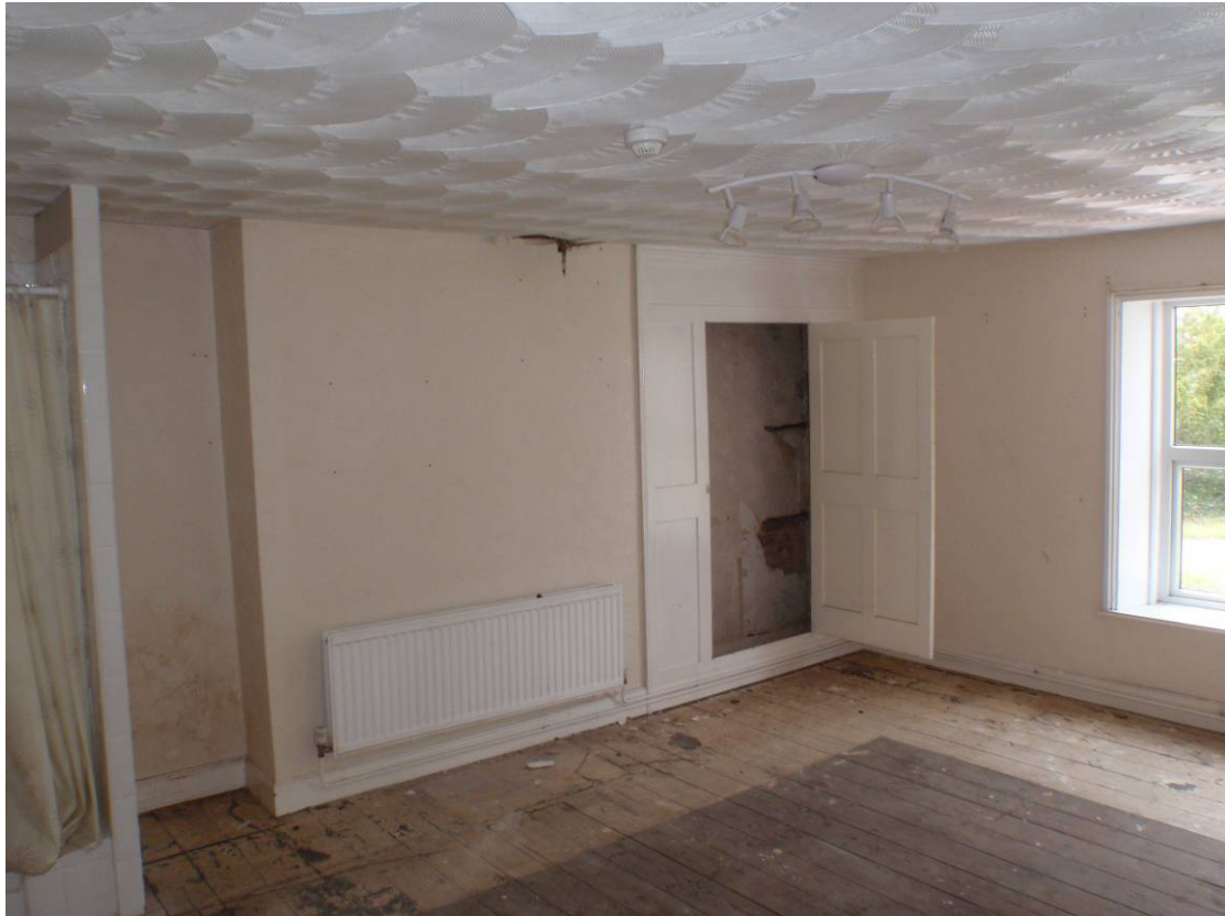
Plate 14 Building 2, upper storey, northern room, looking northeast
