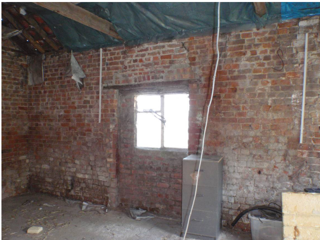
Plate 21 Building 8, interior showing window in blocked doorway, looking south
