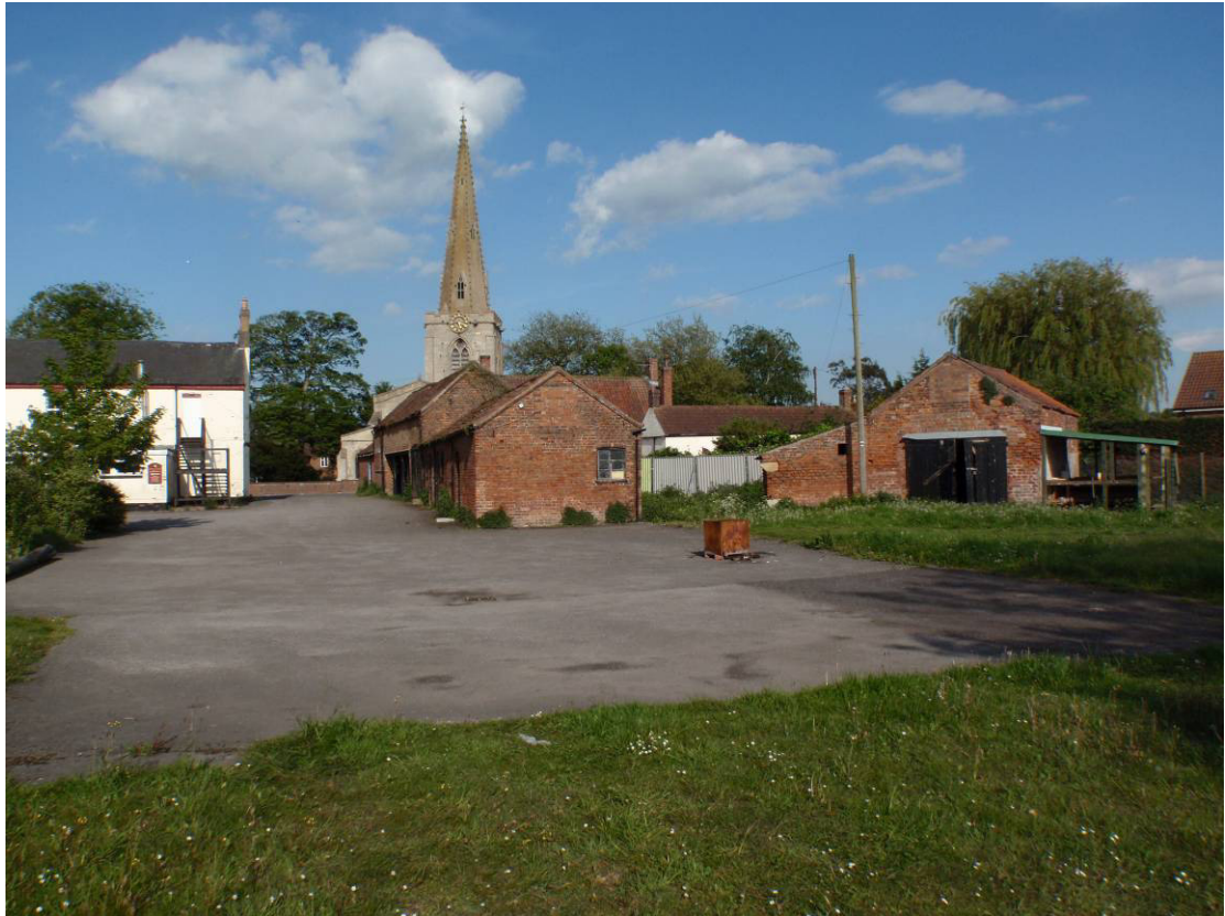
Plate 1 General view of Site from rear (west side), looking east
