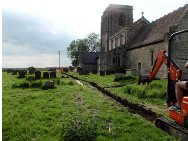
Plate 5 – View of service trench near completion, looking west
