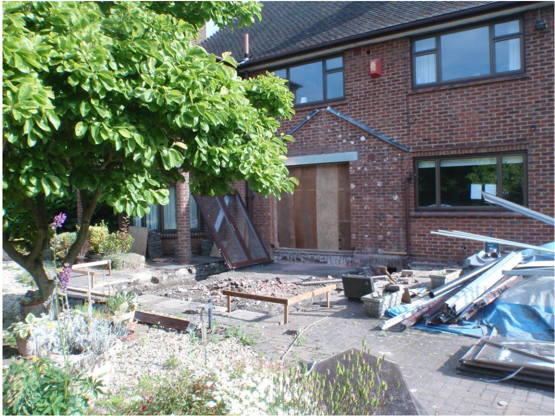
Plate 1. Re-excavated conservatory footings, Area 1, looking north
