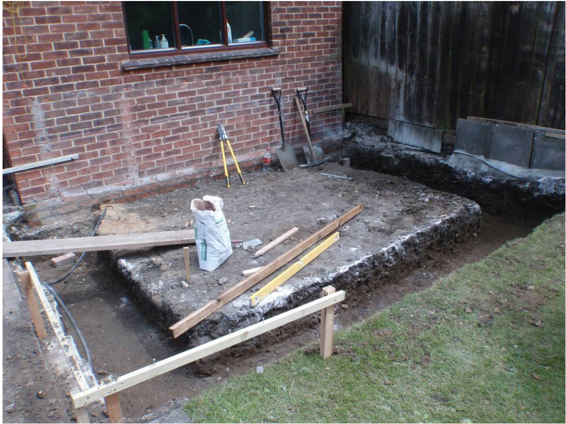
Plate 3. Completed extension footings, Area 2, looking northeast
