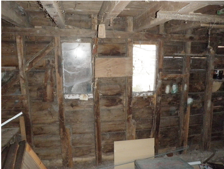
Plate 12. The windows on the northwest wall of Shed A are original and were possibly mirrored on the southeast wall prior to its alteration
