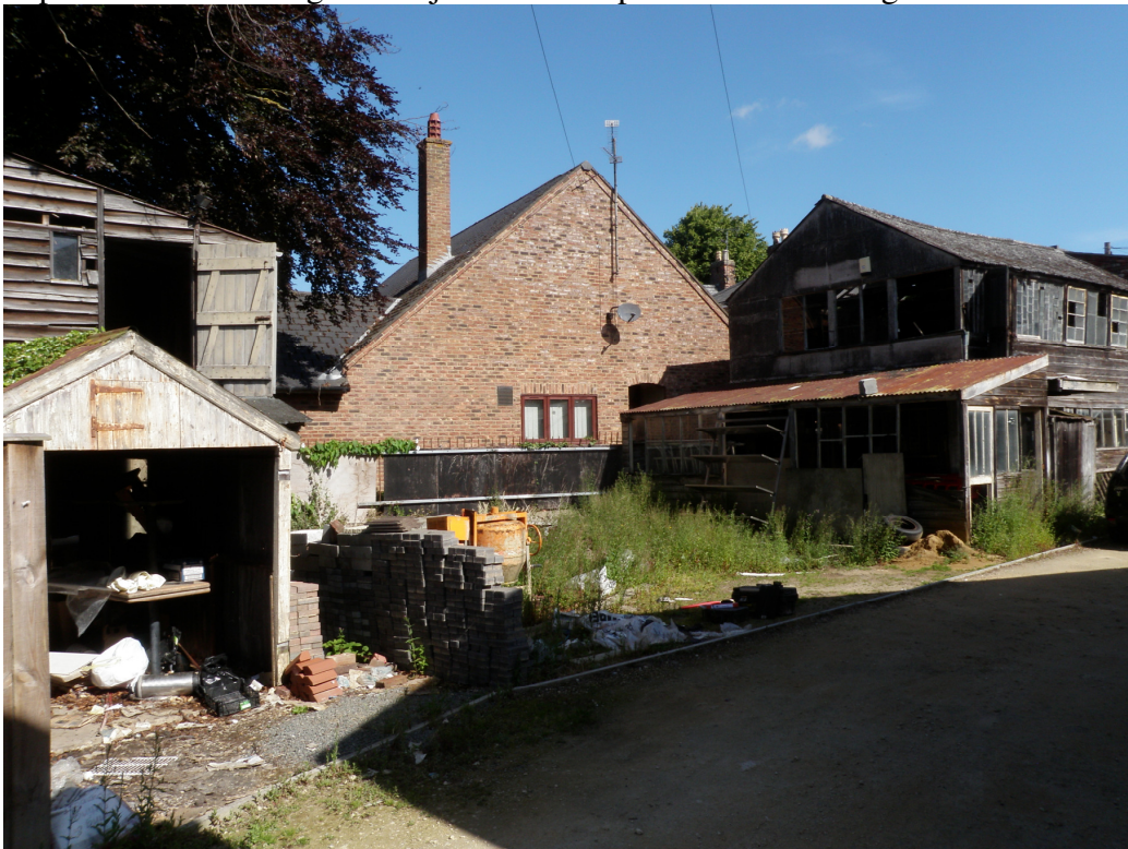
Plate 1. General view of Buildings 1 (left) & 2 (right) looking north from the entrance on Bull Lane.
