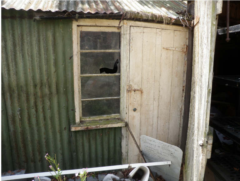
Plate 6. The corrugated iron wall of Shed B with door and window. To the right of the door is 1.45m wide opening allowing free access between the sheds.
