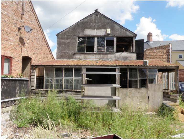
Plate 17. Building 2 Shed B. End view showing its relationship and larger ground floor width compared with Shed A
