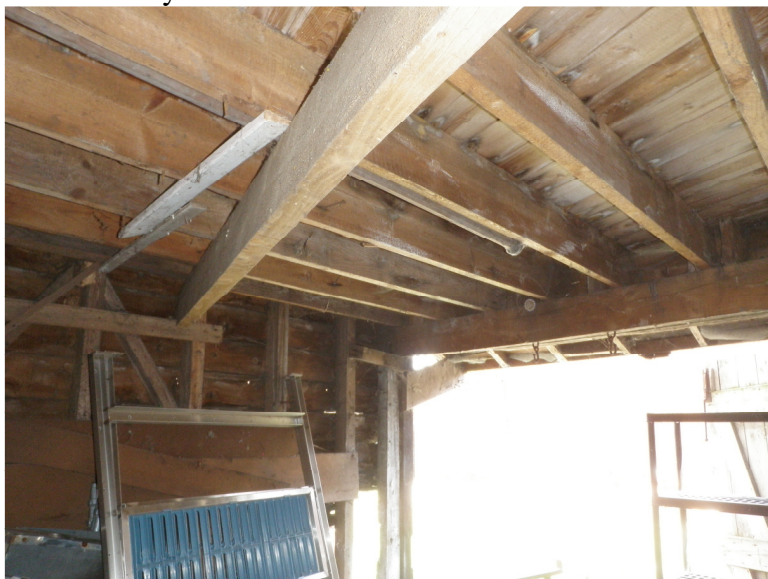
Plate 7. The sturdily constructed interior of Shed C looking towards its entrance. Note the modern timbers that support the first floor that show this structure to be of fairly recent (post-war) construction
