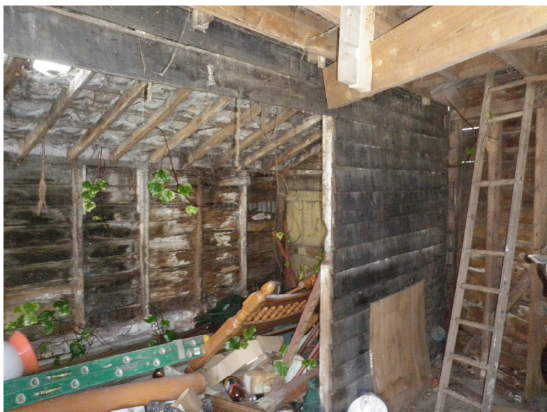
Plate 3. Cut away in northeastern wall showing pantile roof and previously external timbers
