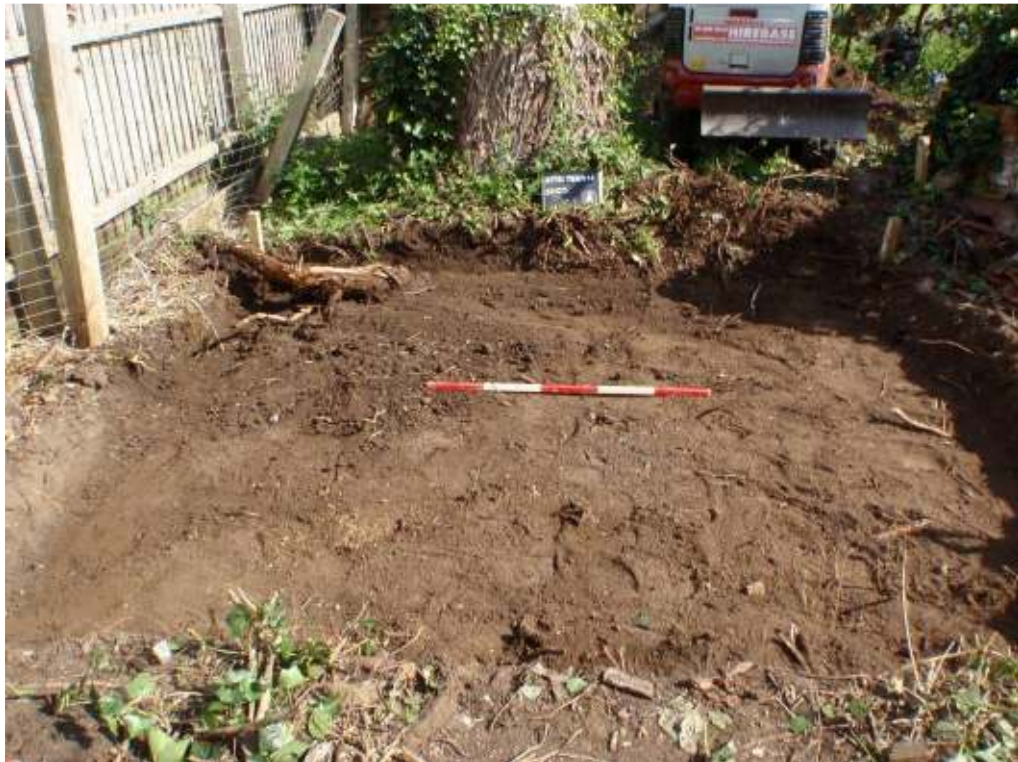
Plate 2. Site looking north following topsoil strip
