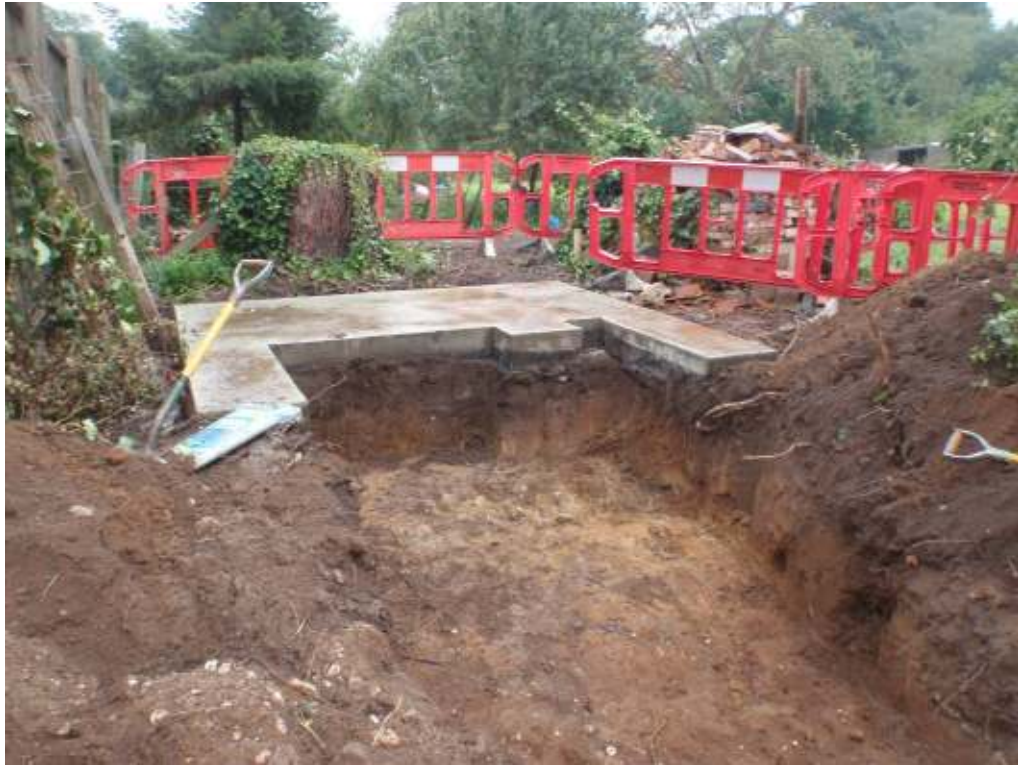
Plate 3. General view of service access excavation looking northeast
