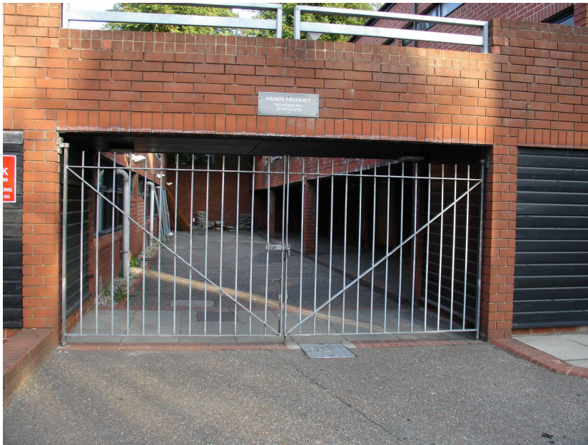
Plate 4 - The gated yard beneath the 1970s flats with walkway over, looking east
