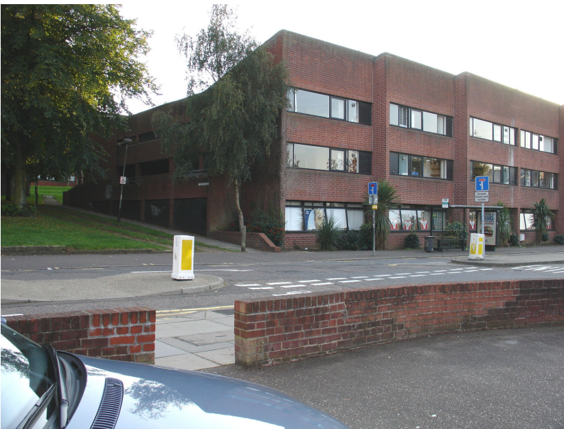
Plate 2 - View showing the 1970s flats with the rise in ground level along St. Benedict's Alley, looking southwest
