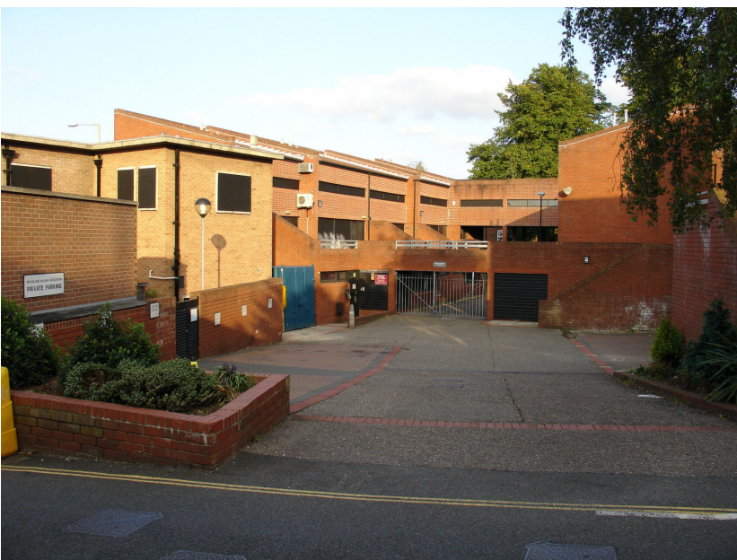
Plate 3 - The open yard showing the drop in height, looking east from Wellington Lane
