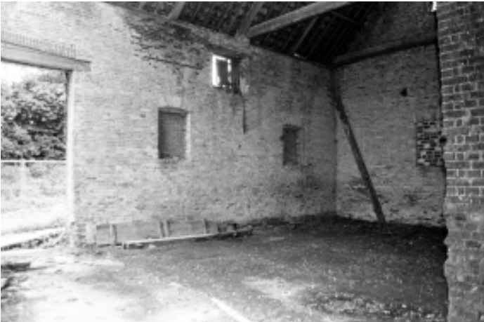
Plate 28 Barn Interior, southern part of east wall, showing blocked ventilator windows and pitching hole above, looking southeast
