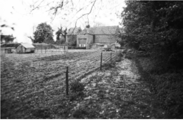
Plate 1 General View of Barn, from River Stiffkey, looking east
