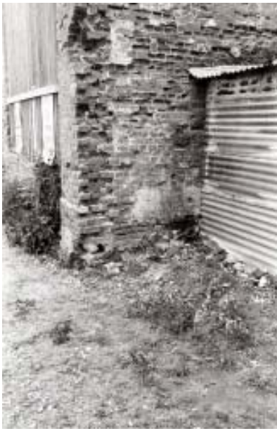
Plate 11 Porch, south side, showing flint cobble foundation and scar of removed wall, looking northeast
