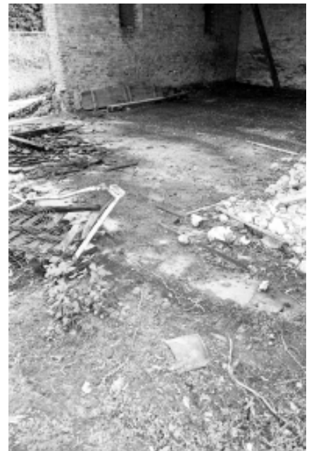
Plate 20 Concrete Floor and Brick Edging, Central Bay, looking southeast
