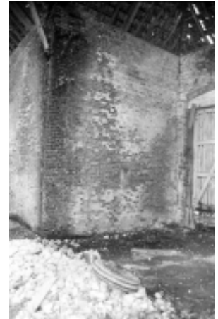
Plate 27 Porch Interior, south wall, showing alcove, looking southwest
