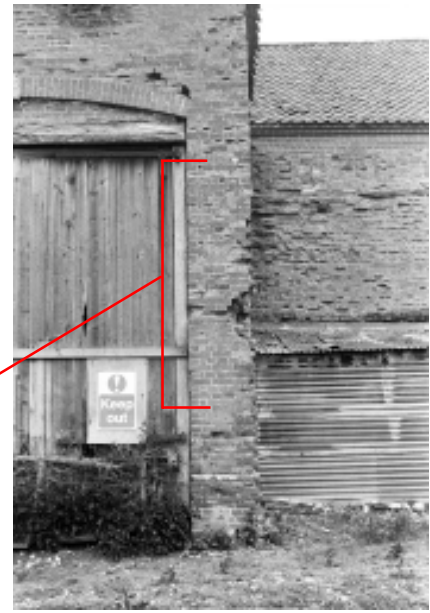
Plate 12 Porch, Western Elevation, showing positions of inscribed bricks, looking east
