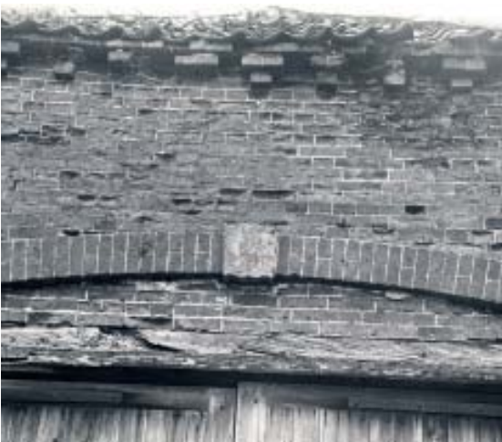
Plate 9 Western Elevation of Porch, showing arch, keystone and dentil eaves, looking east
