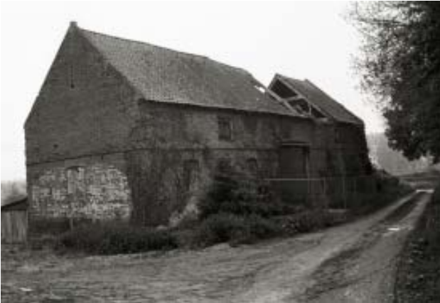
Plate 2 South and East Elevations of Barn, looking north
