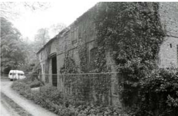
Plate 3 South Elevation, showing blocked ventilator window and breather slit, looking northeast
