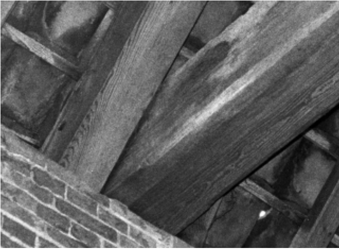
Plate 21 Chamfered Beam, detail, looking southeast
