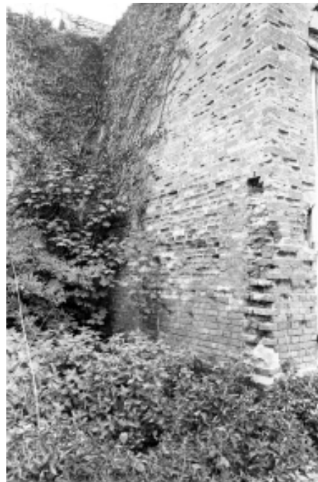
Plate 15 Porch, north side, showing scar of removed wall, looking southeast
