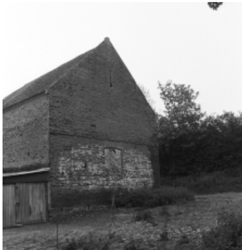
Plate 3 South Elevation, showing blocked ventilator window and breather slit, looking northeast
