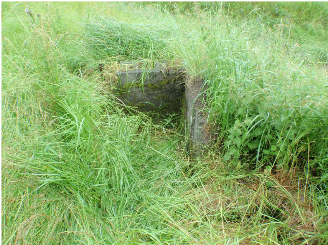
Plate 24. Asset 189 Tetney, zig-zag wall fragment looking northeast
