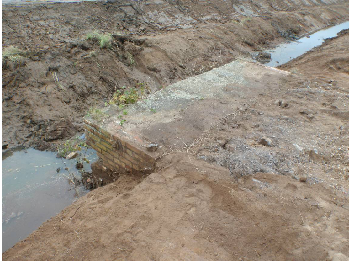
Plate 19. Asset 178. Bridge footing [015], Section 4, looking northwest
