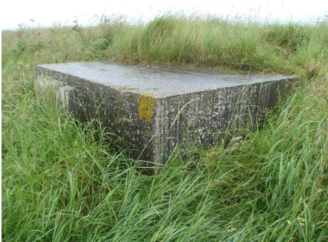
Plate 25. Asset 206/7 Tetney, pillbox looking south
