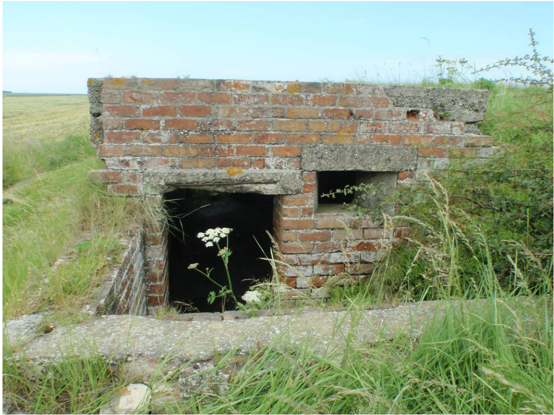
Plate 5. Asset 167, south entrance of infantry house, Elevation 2, looking NNW
