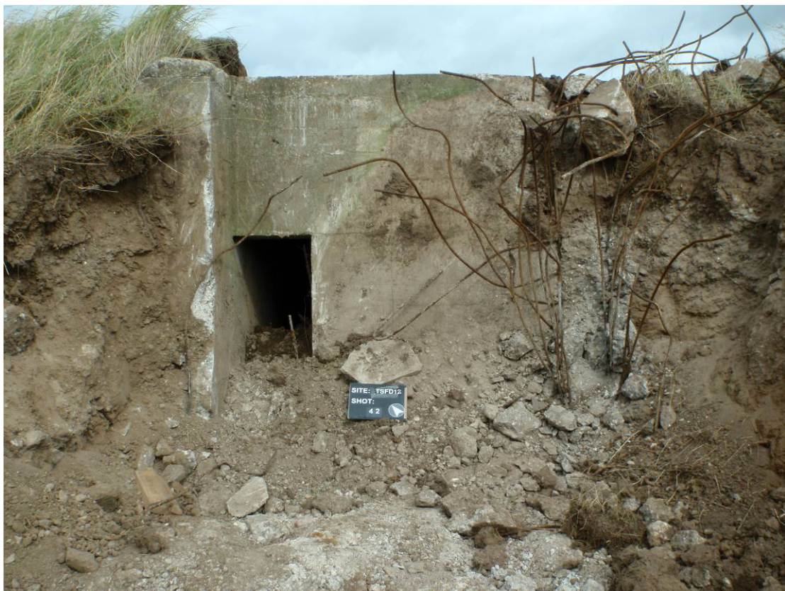
Plate 26. Asset 206/7 landward opening, Section 11, looking northeast
