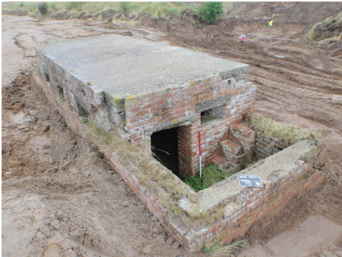
Plate 10. Asset 167 after removal of vegetation, looking north
