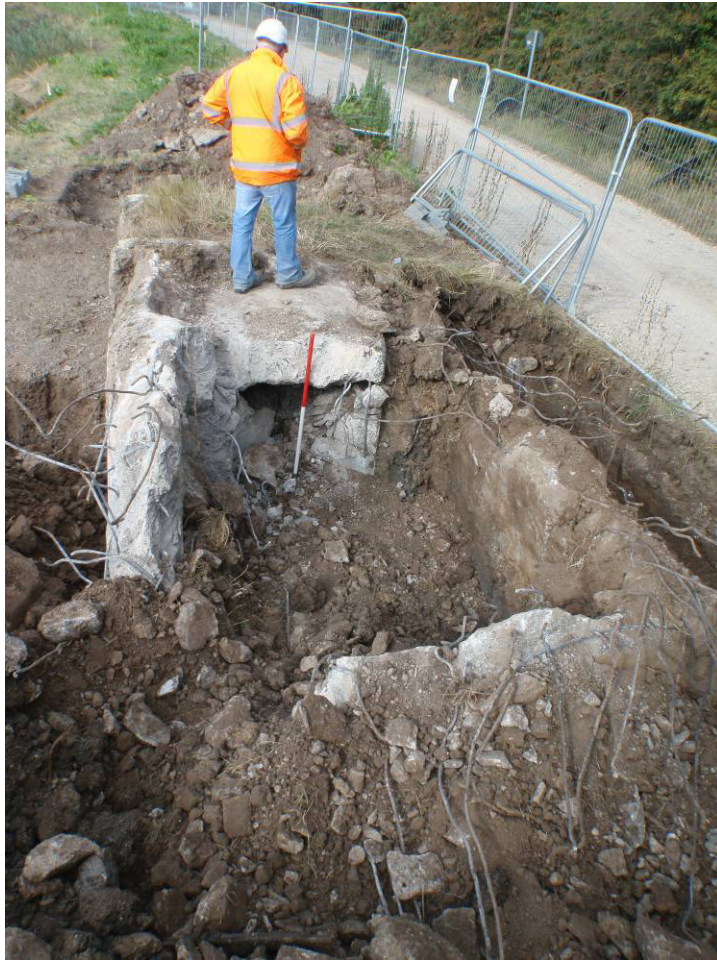
Plate 3. Asset 81 part demolished, looking west
