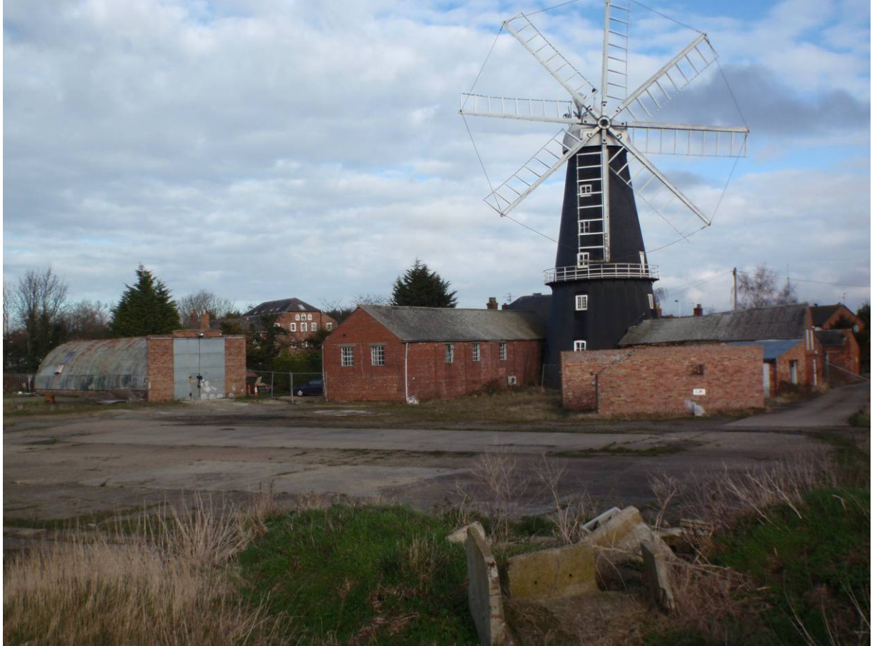
Plate 2. Mill complex, looking northeast, showing attached granary and brewery with the Nissen hut to the left, further to the north
