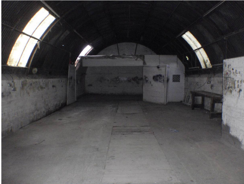
Plate 16. Interior of the Nissen hut, looking north toward the partitioned area used as a spray booth
