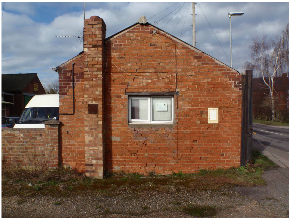
Plate 11. South facing gable of bakehouse with modern brickwork in verge, additional chimney stick and trefoil decoration in apex of roof
