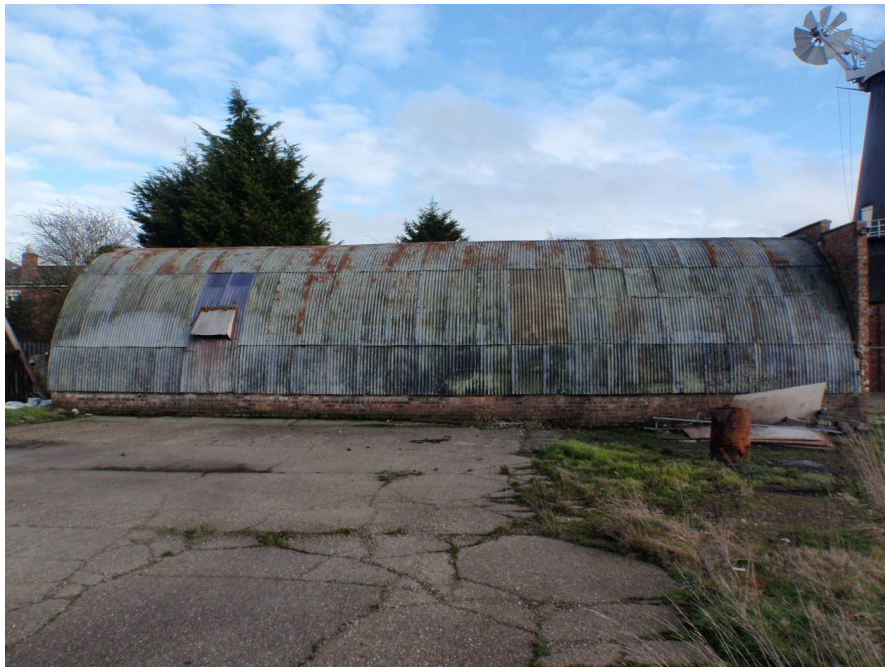
Plate 14. The Nissen hut, looking east, noting the projecting elevation to the right and the flush gable to the left.
