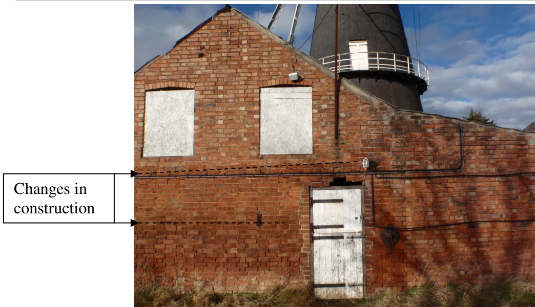
Plate 17. The Granary. South elevation showing several phases of construction
