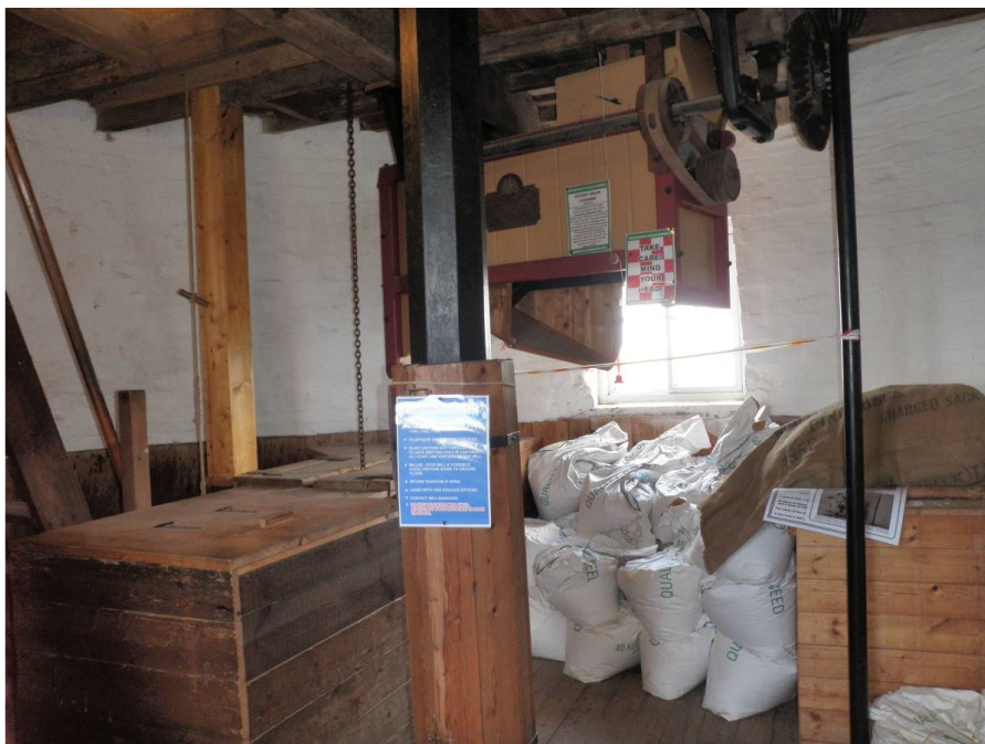
Plate 6. The Lower Bin floor with raised sack traps for ease of handling
