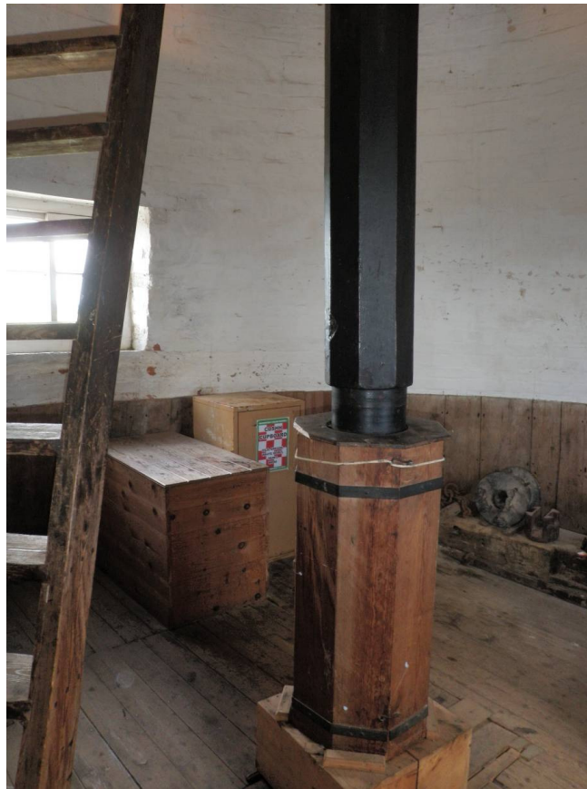
Plate 5. The Upper Bin floor with partially boarded walls
