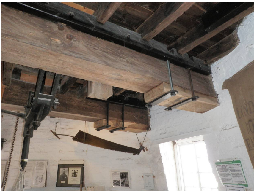
Plate 8. The Meal Floor. The beams supporting the stone floor
