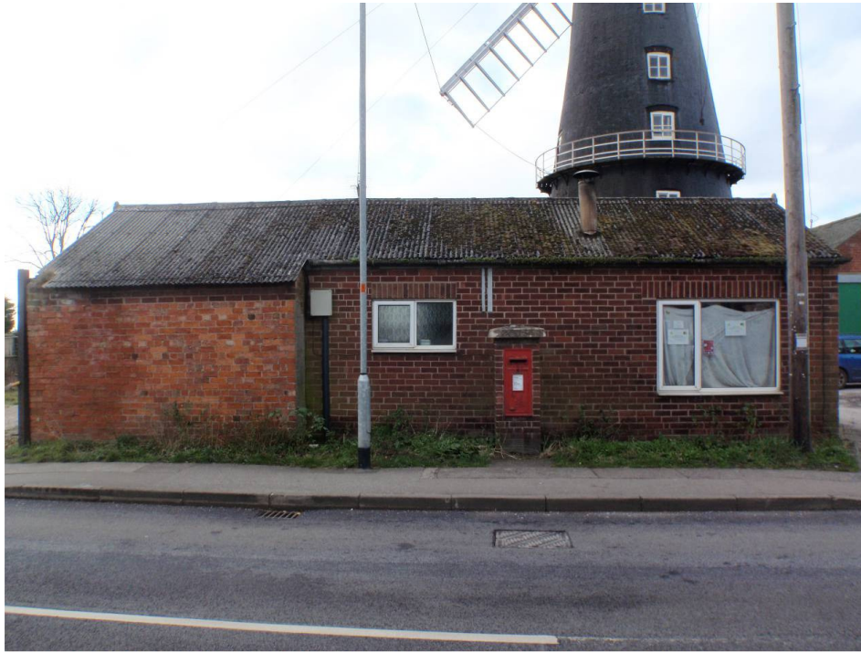
Plate 10. Eastern elevation of bakehouse showing two distinct construction phases
