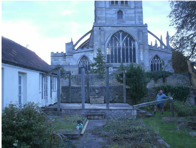
Plate 1. The site before the groundworks, showing the raised area at the east end. Looking east south-east
