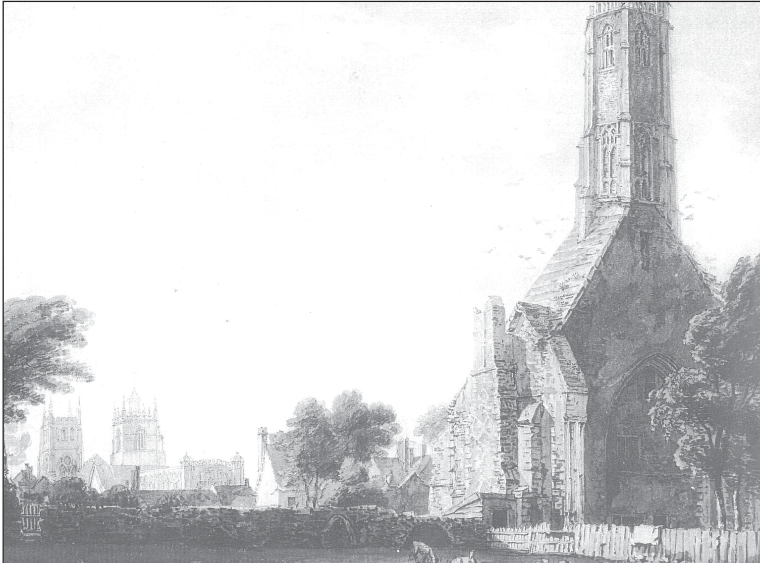
Figure 4 - Thomas Hearne's view of Greyfriars' tower, late 18 th century. The infilled chancel arch is visible with three floors represented. A possible portion of the north chancel wall also survives (right). Also visible is the archway of the Chapter House door (centre) and a second arch to the right. Note also the Tudor diaper brickwork on the chimney stack butting the tower.
