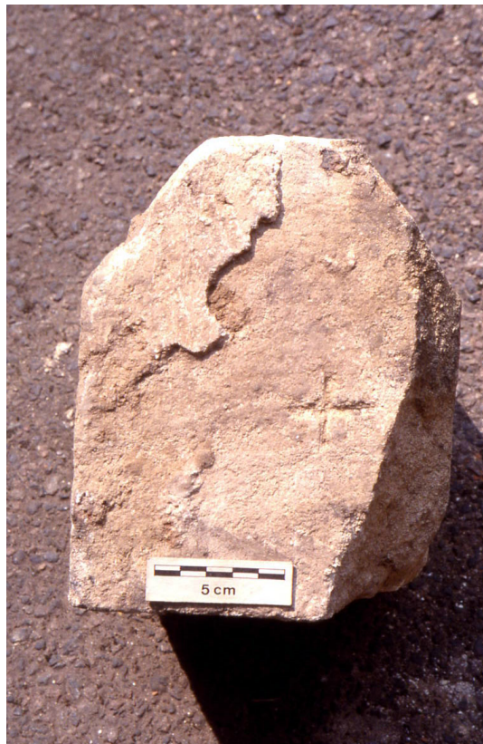
Plate 32 - Incised cross on bedding joint of voussoir rib
