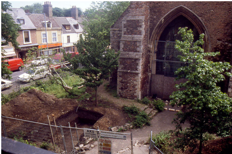
Plate 2 - View of Trench 1 during excavation, looking northeast
