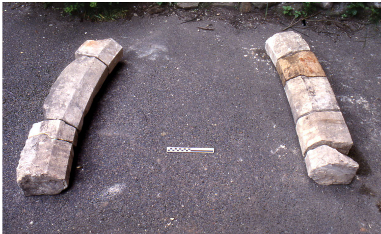
Plate 31 - Vaulting ribs from (505) showing the curvature of the voussoirs
