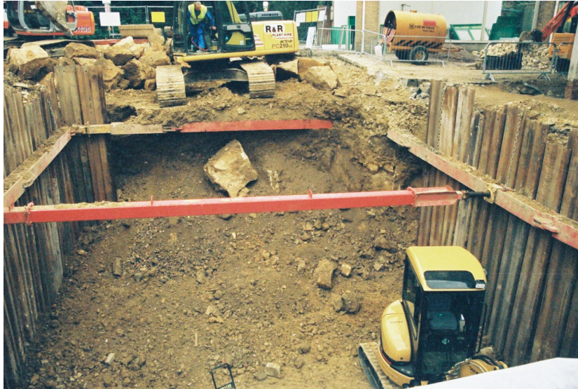
Plate 1 - View showing the excavated trench for the new storage tanks
