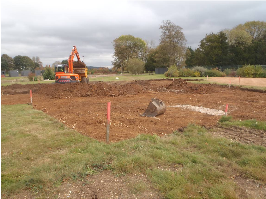
Plate 4 – Working shot of house footprint being stripped, looking southeast
