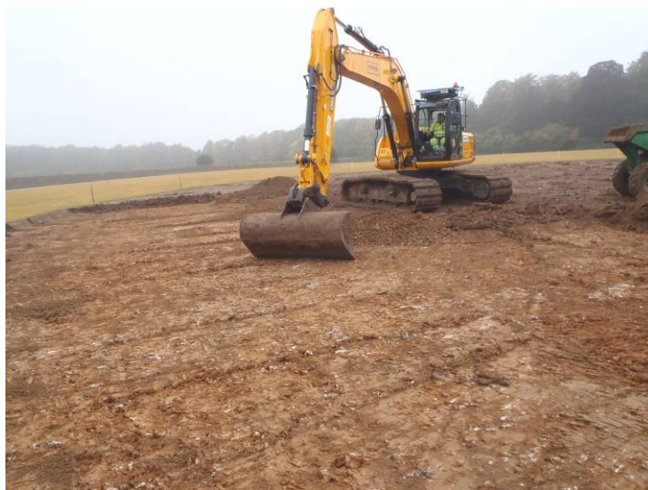
Plate 2 – Working shot of Pond Area, looking northwest
