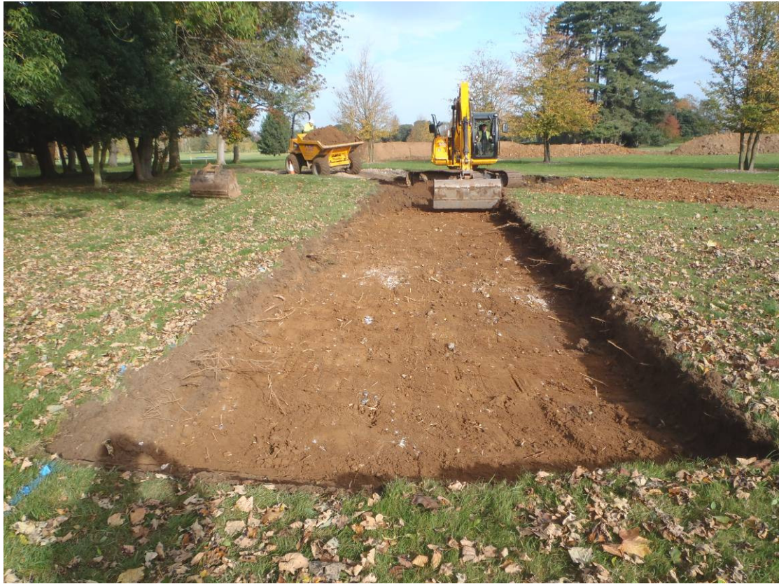
Plate 6 – Stripping northern section of Road B, looking north
