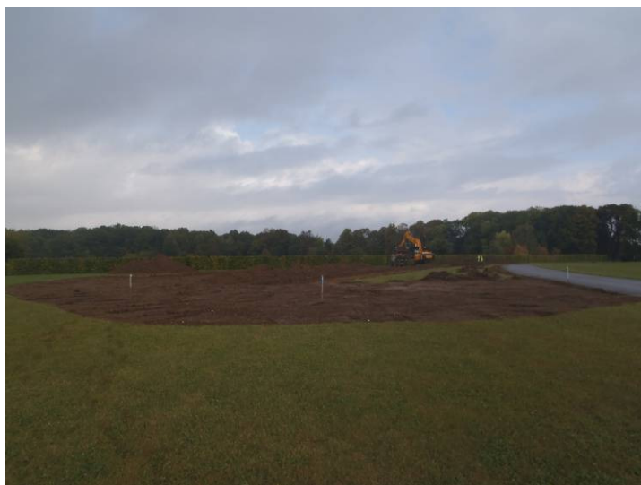
Plate 3 – Working shot of Mound Area A, looking north
