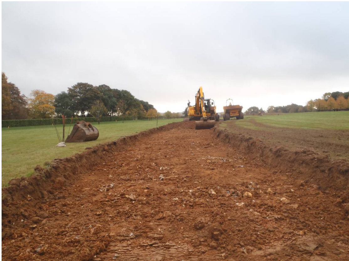
Plate 5 – Stripping of main section of Road A, looking south
