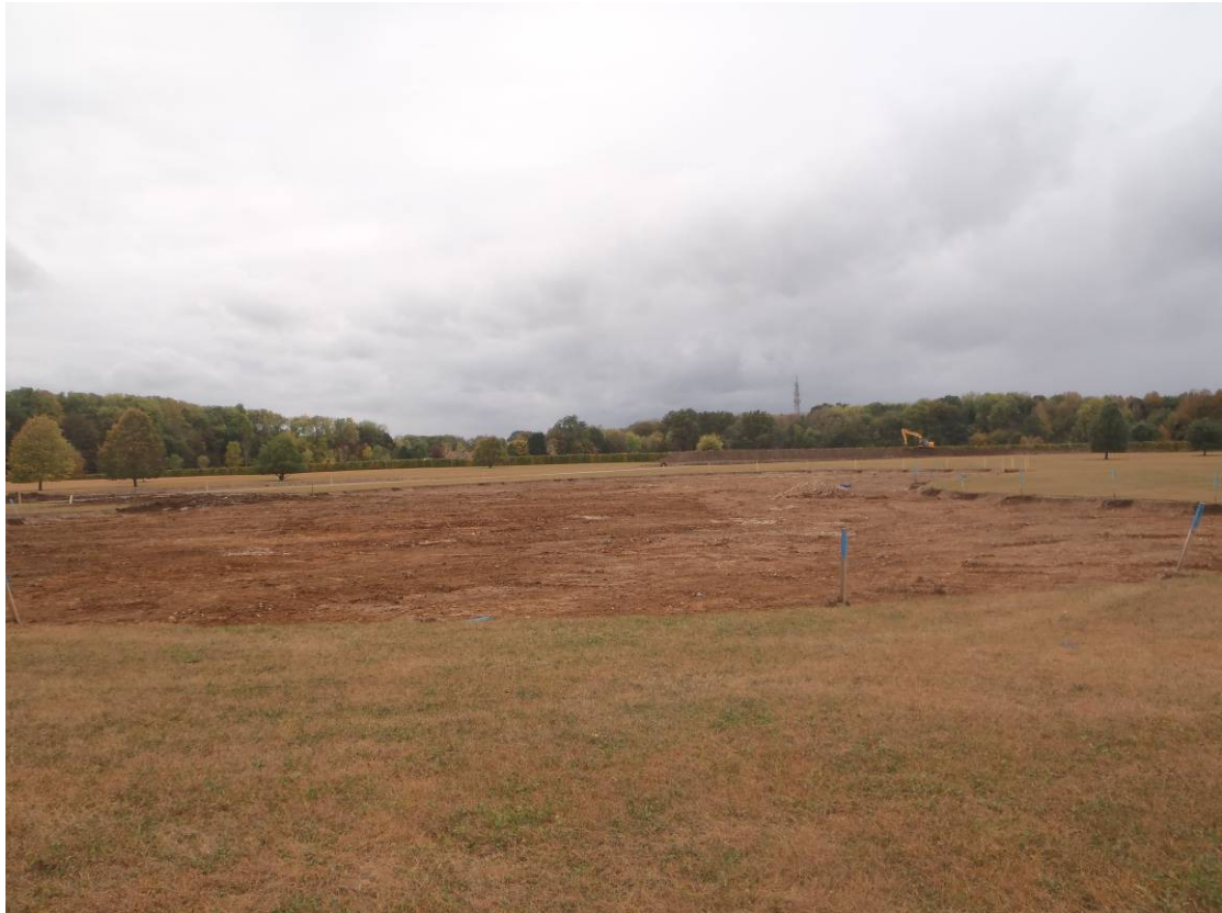
Plate 8 – Pond Area fully stripped, looking northwest
