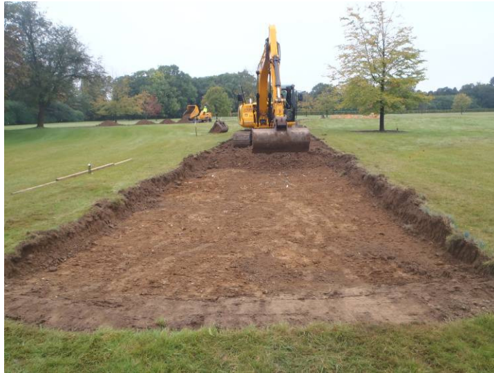
Plate 1 - Working shot of northern end of Road A, looking northwest
