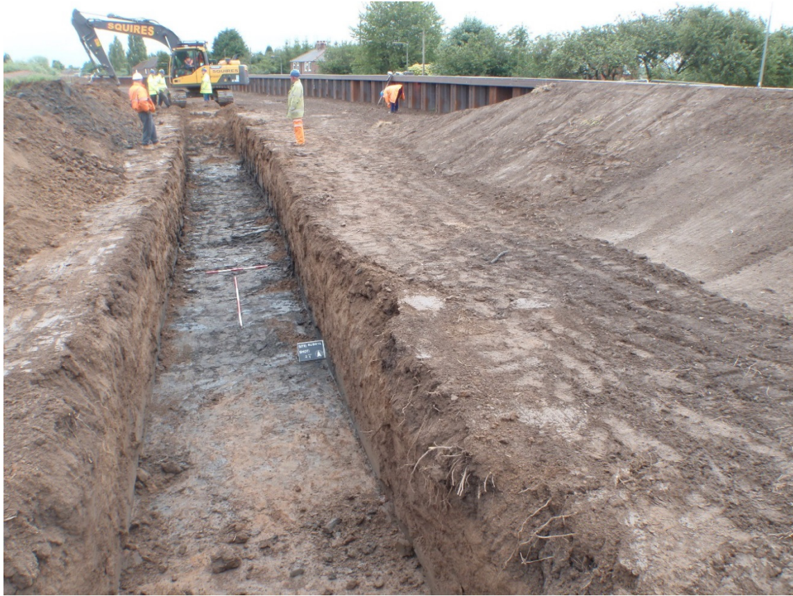
Plate 3. Trench across the warping drain looking north
