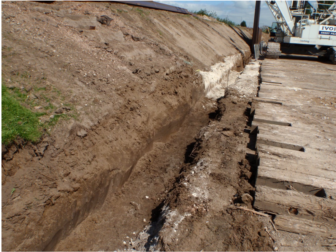
Plate 1. Excavating the footing trench for the flood defence barrier looking north
