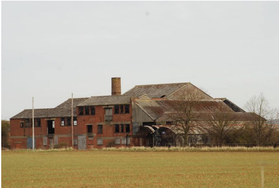
Plate 1. General view of the south and west elevations of the processing area of the flax factory.
