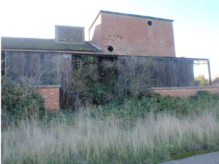
Plate 13. The northern end of the east elevation showing the corrugated iron lean-to structure. Looking northwest
