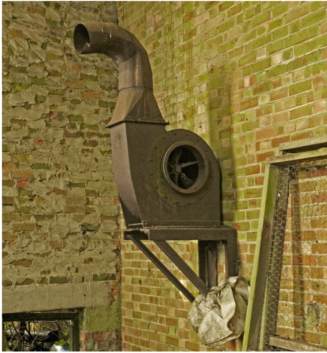
Plate 19. Part of a centrifugal fan used for dust extraction during the de-seeding process.
