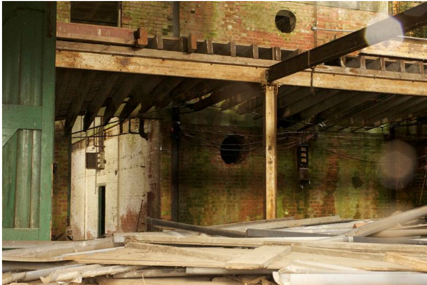
Plate 8. Southern elevation from within the lean-to structure. Looking northeast
