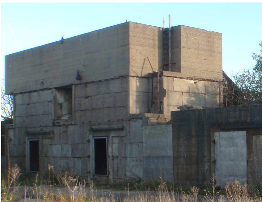
Plate 16. Detail of the retting tanks showing the main tank at the east of the structure. Looking southeast
