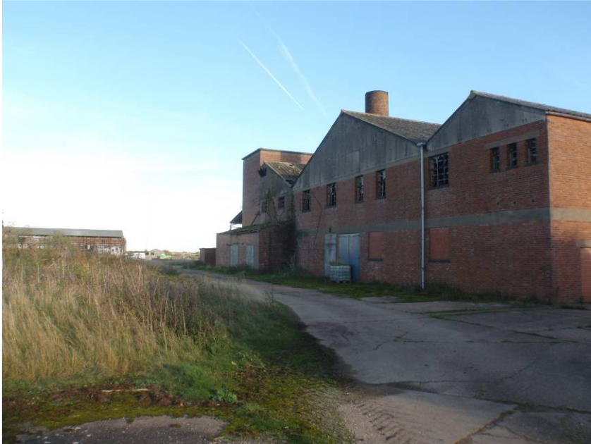
Plate 11. The north elevation showing the boiler chimney. Looking southeast
